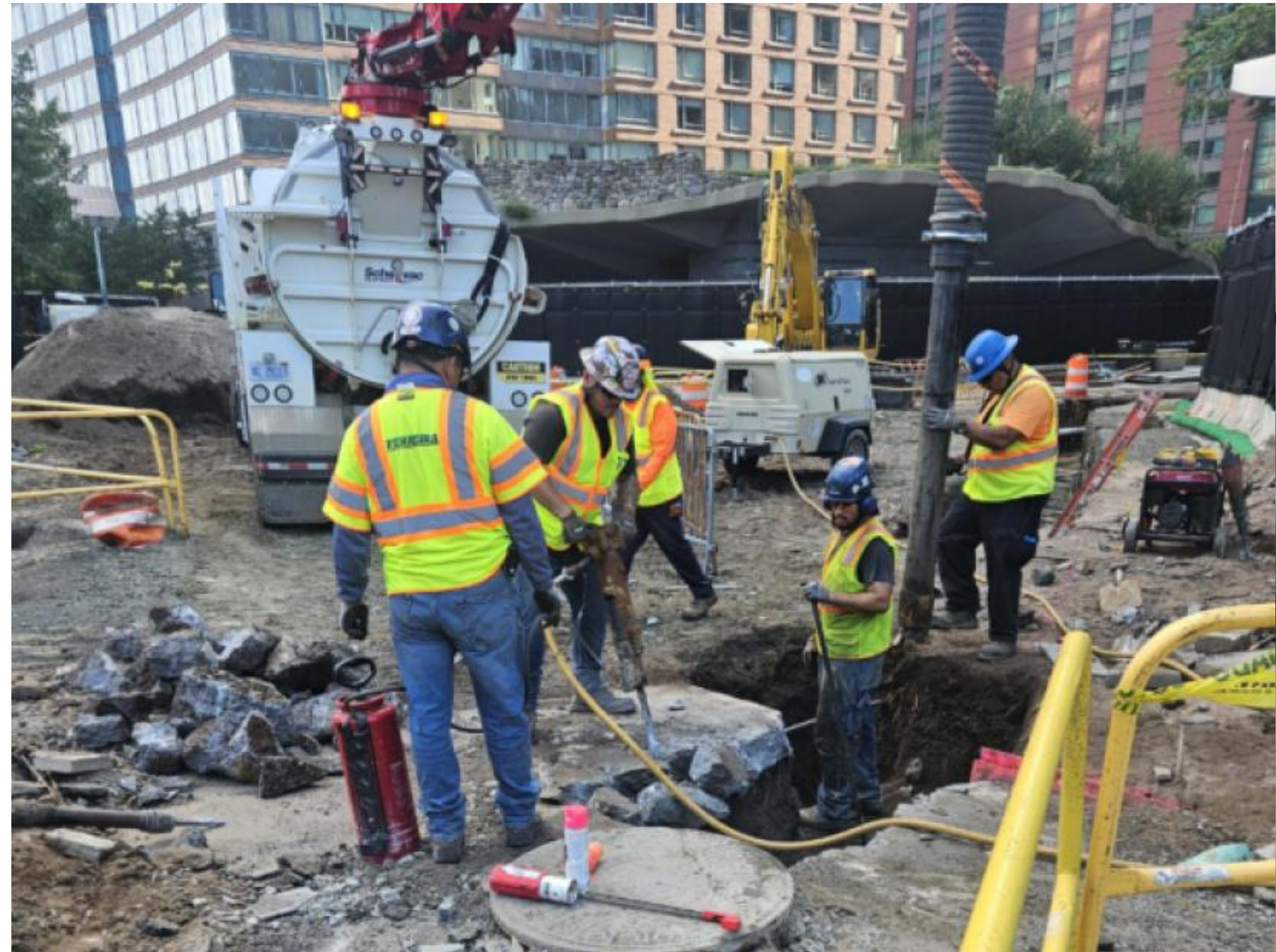
Excavation for electrical ductbank
