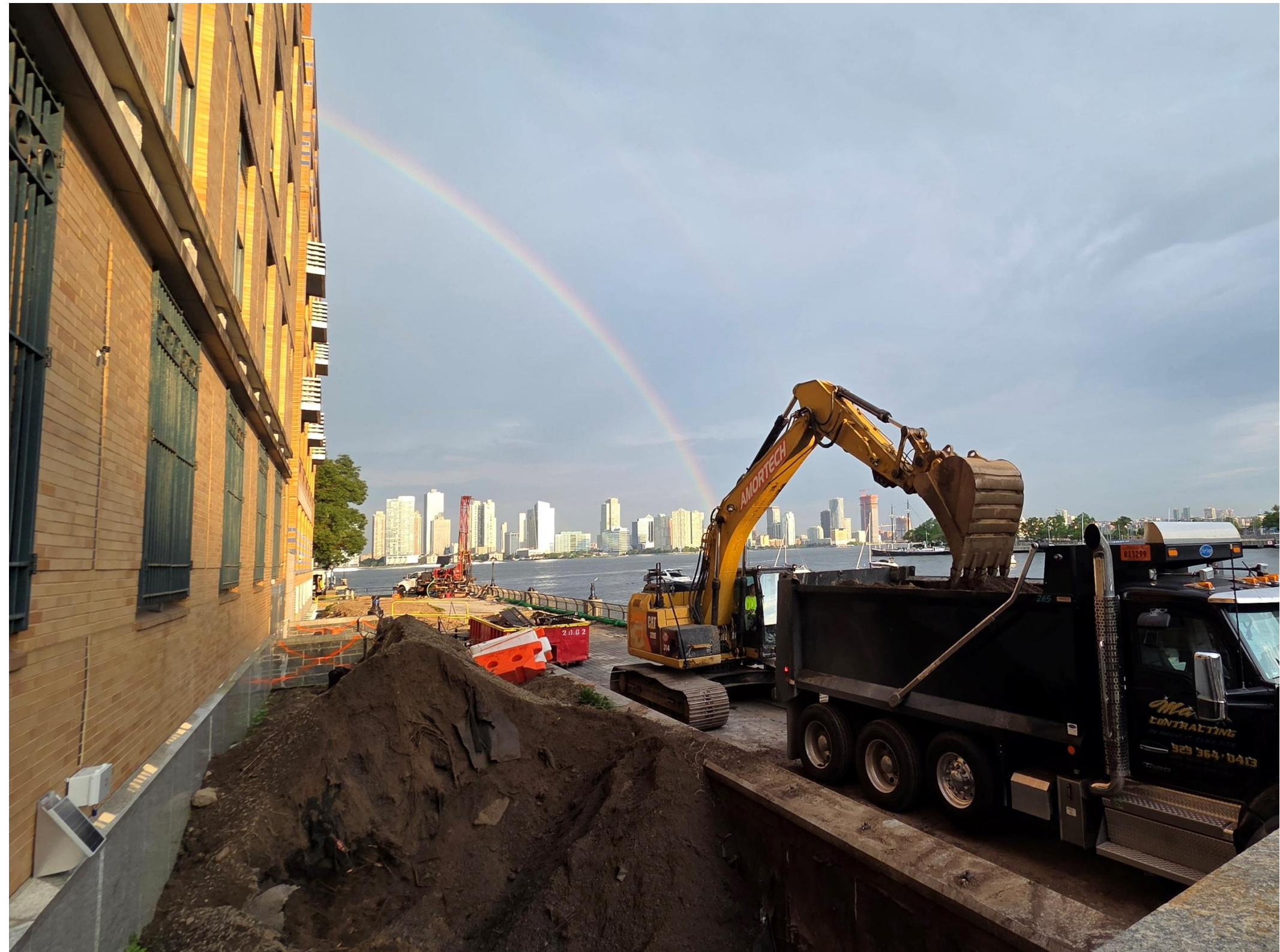
Surface demolition along North Esplanade
