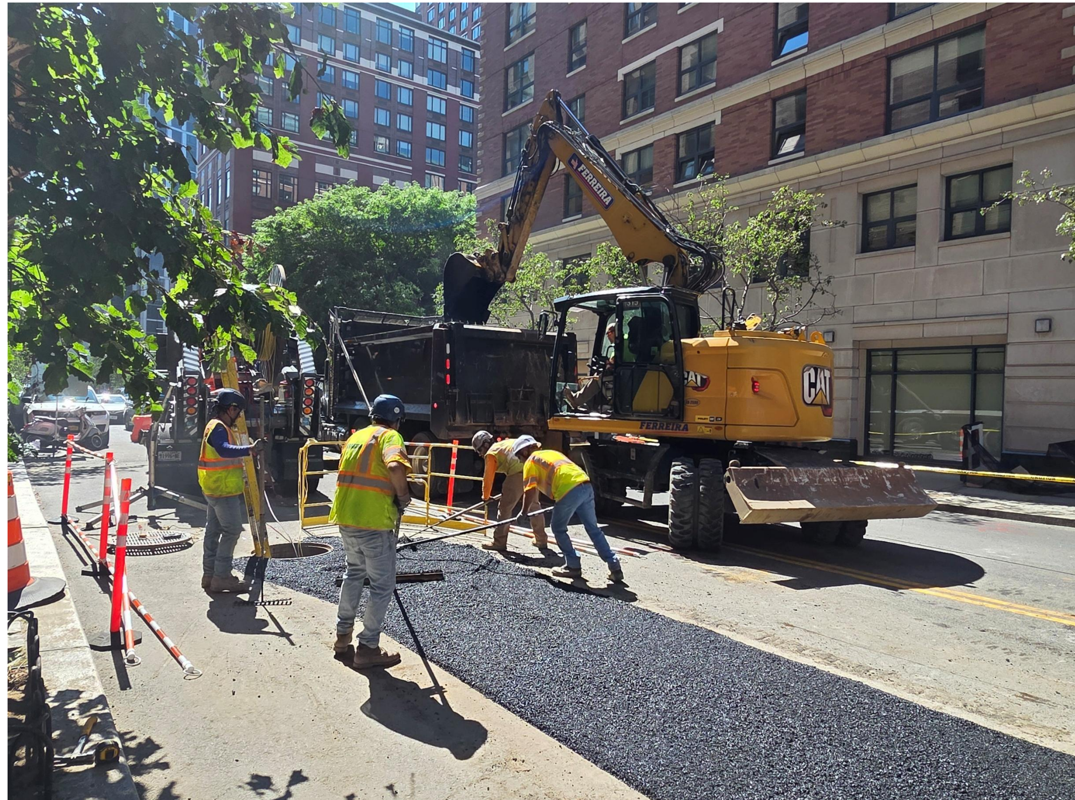
Repaving after the watermain relocation
