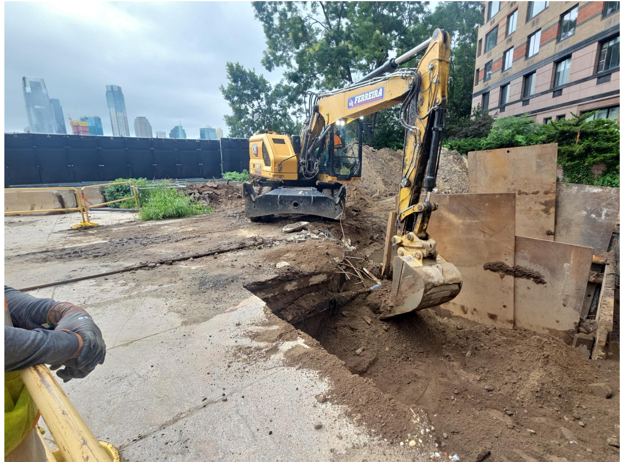
Test pit at tide gate location
