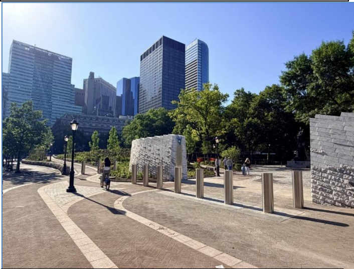
Stone floodwall and bollards
