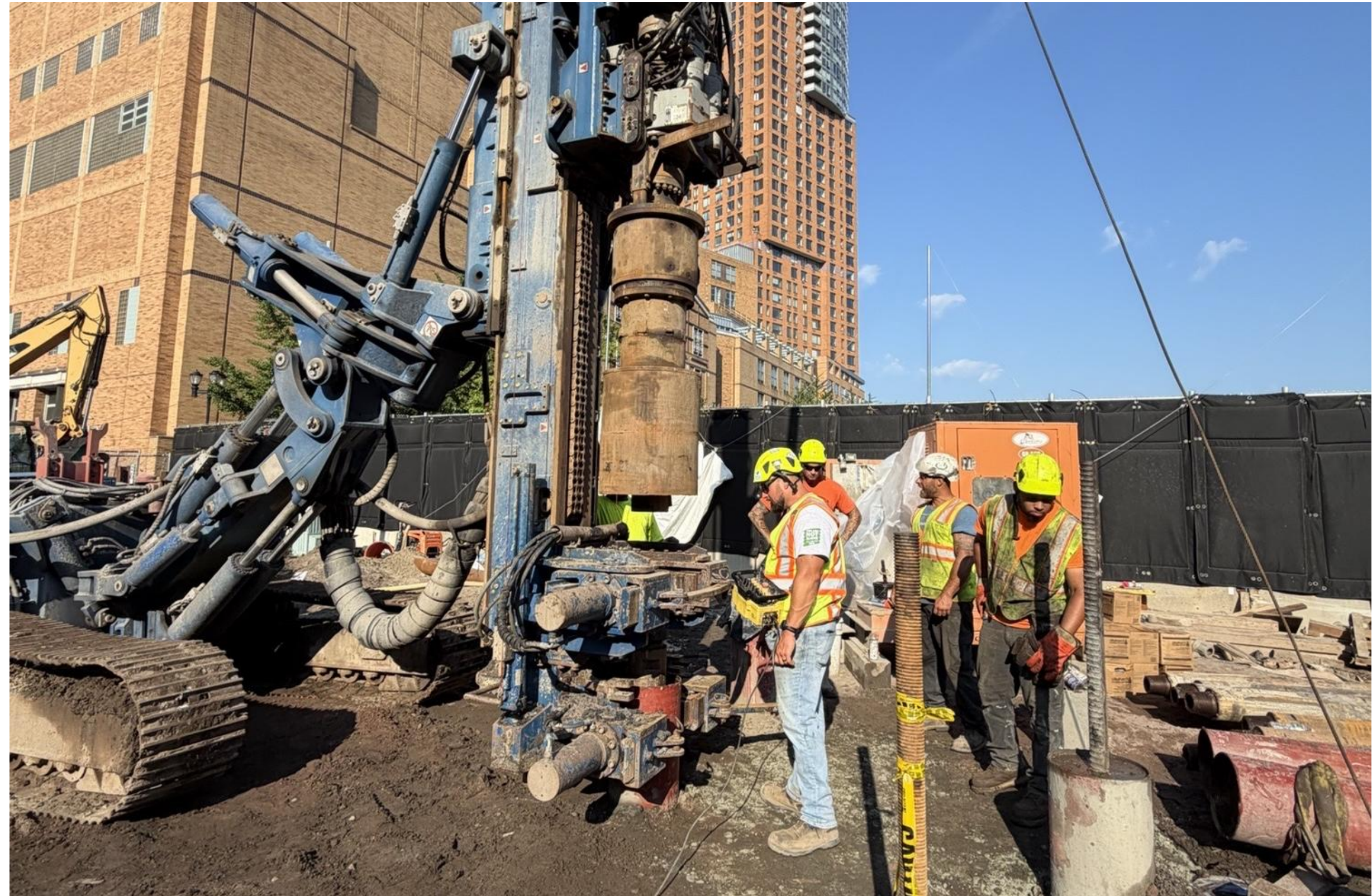
Pile Installation along Route 9A
