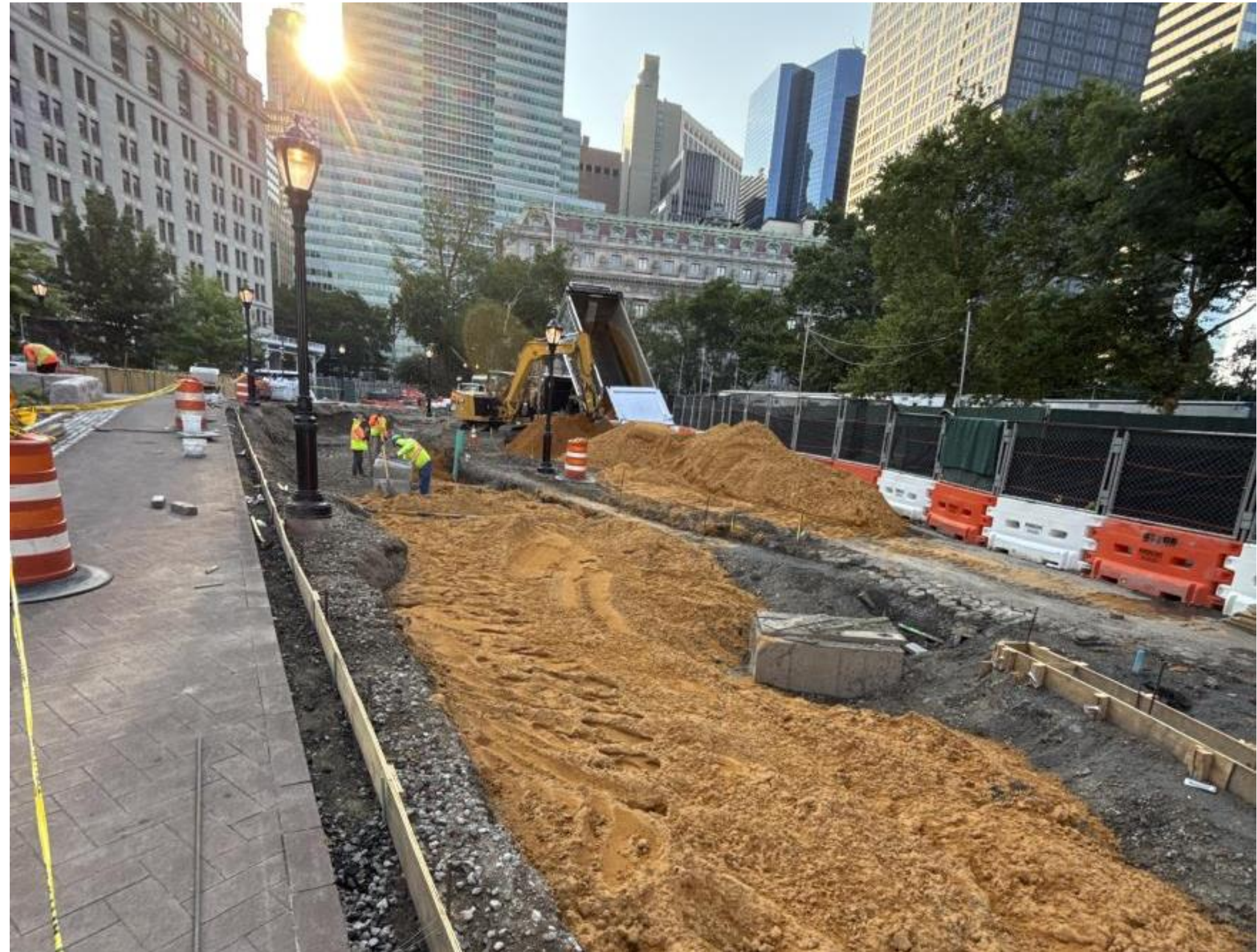
Battery soil installation
