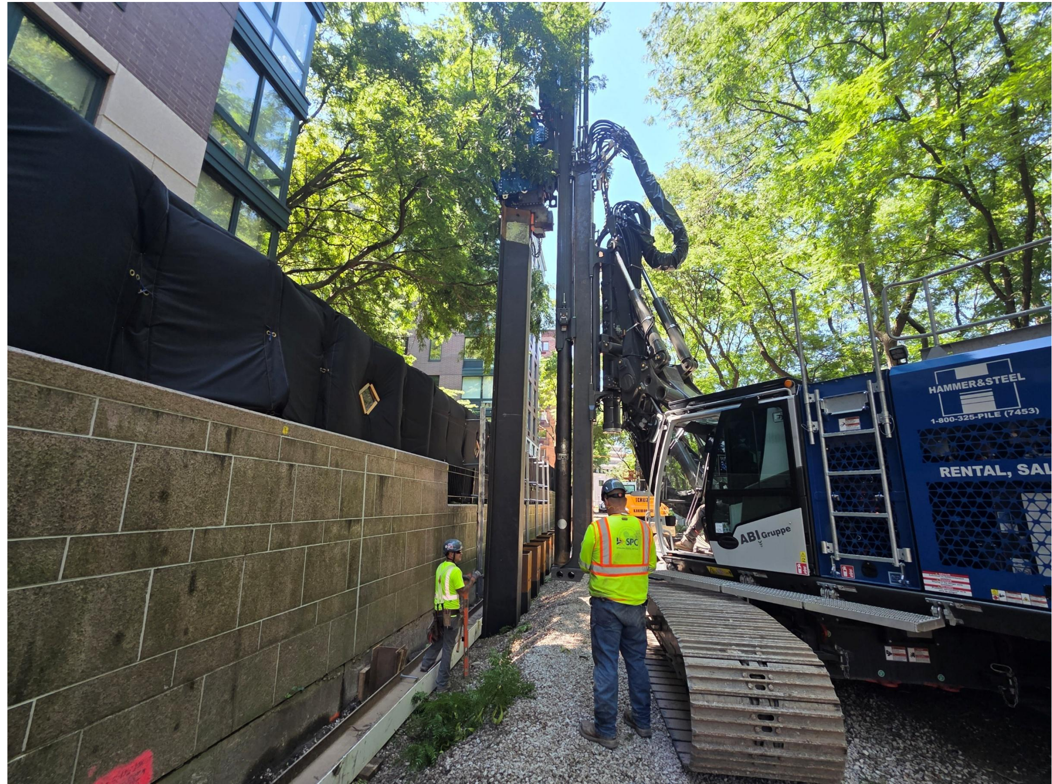
Sheet pile installation along Riverwatch
