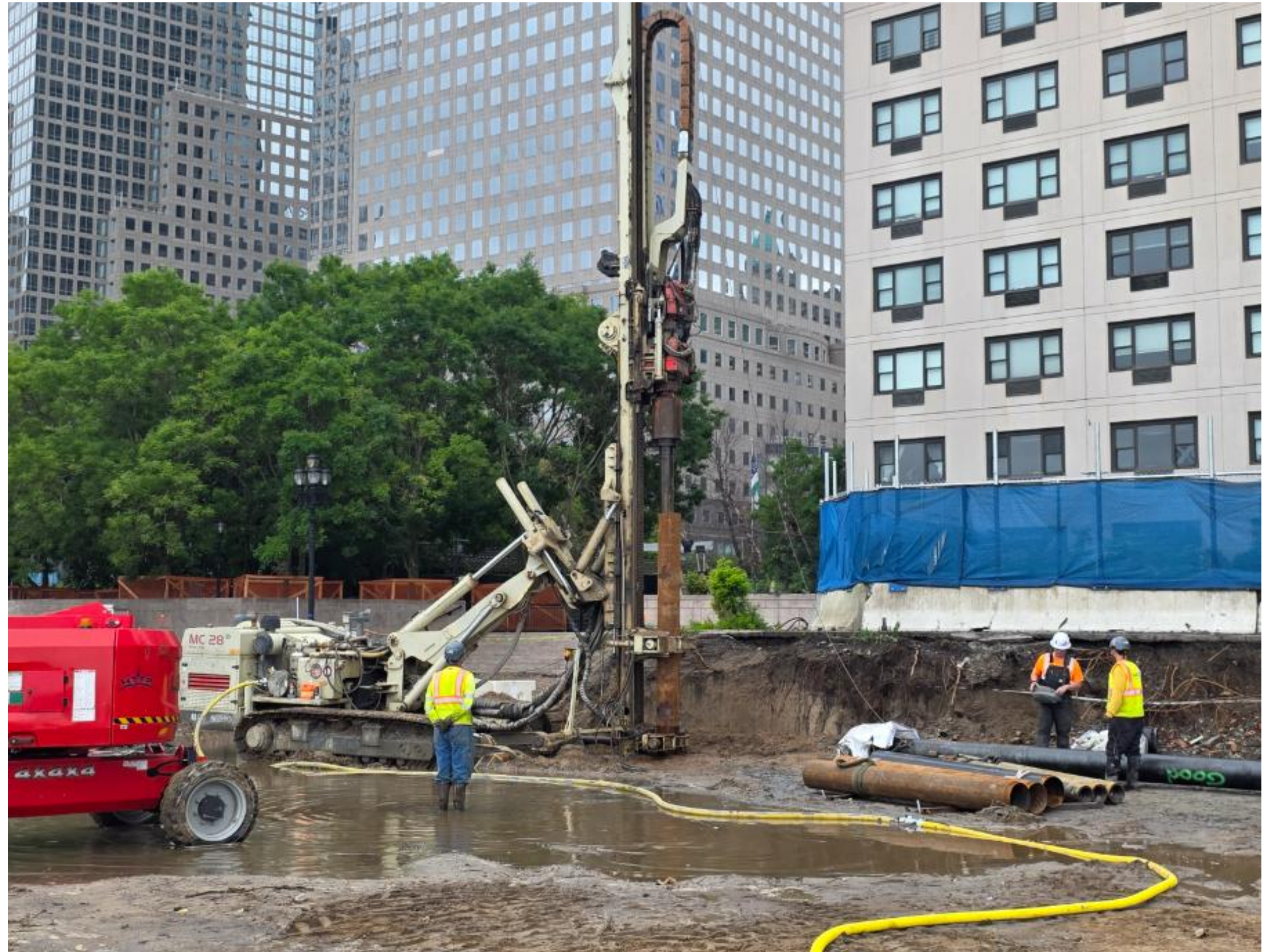
Pile installation at Gateway Plaza
