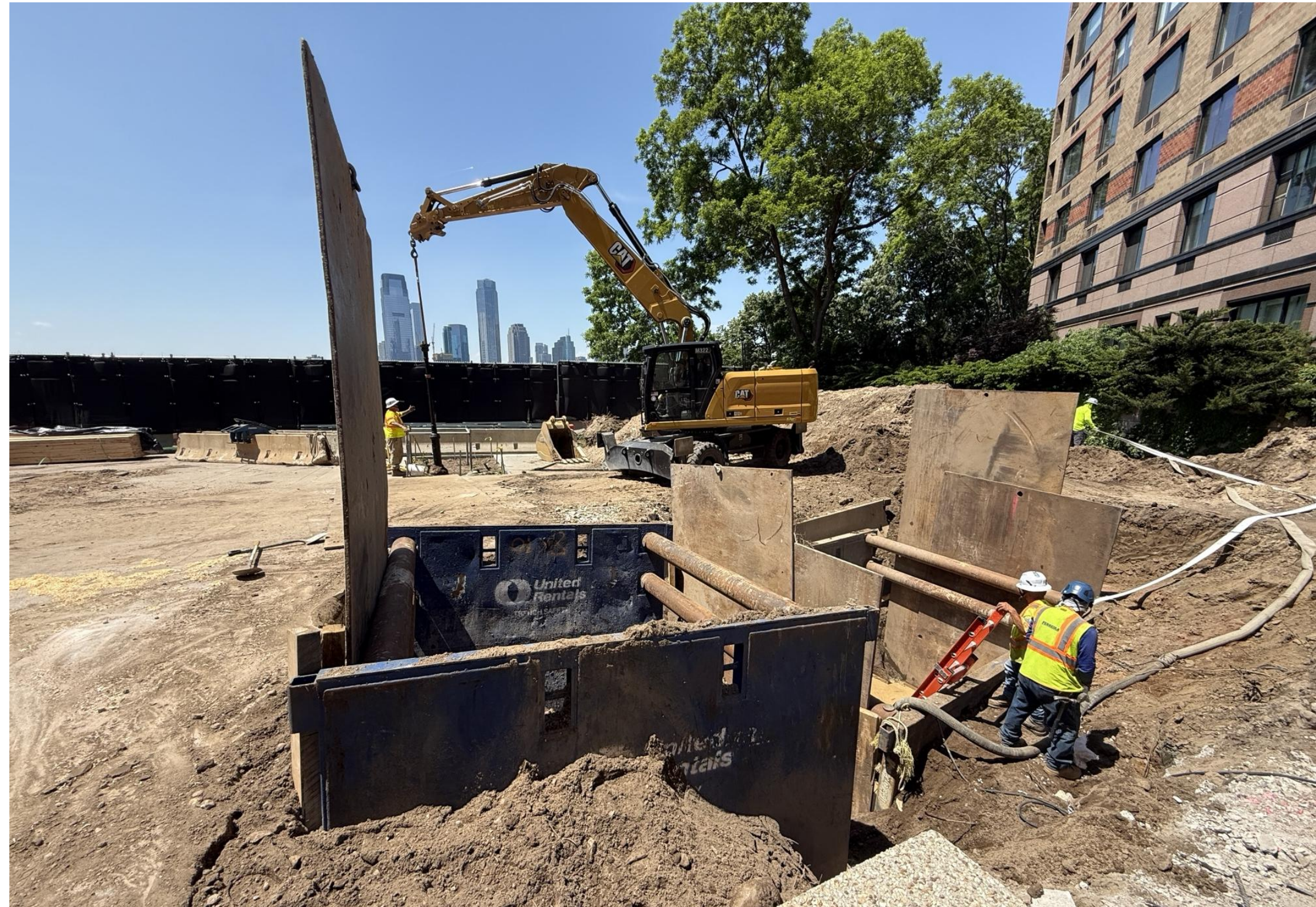
Test pit to identify subsurface utilities at tide gate location
