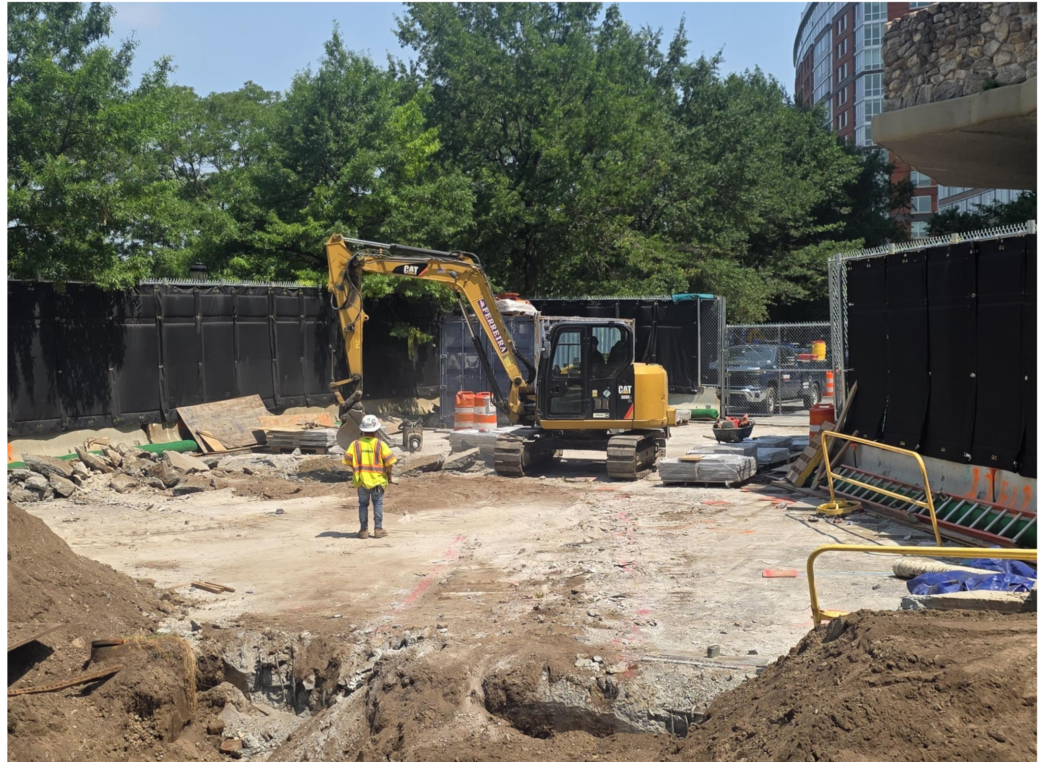
Surface demolition and salvage underway
