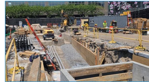
Trench for new ECS ductbank by Winter Garden
