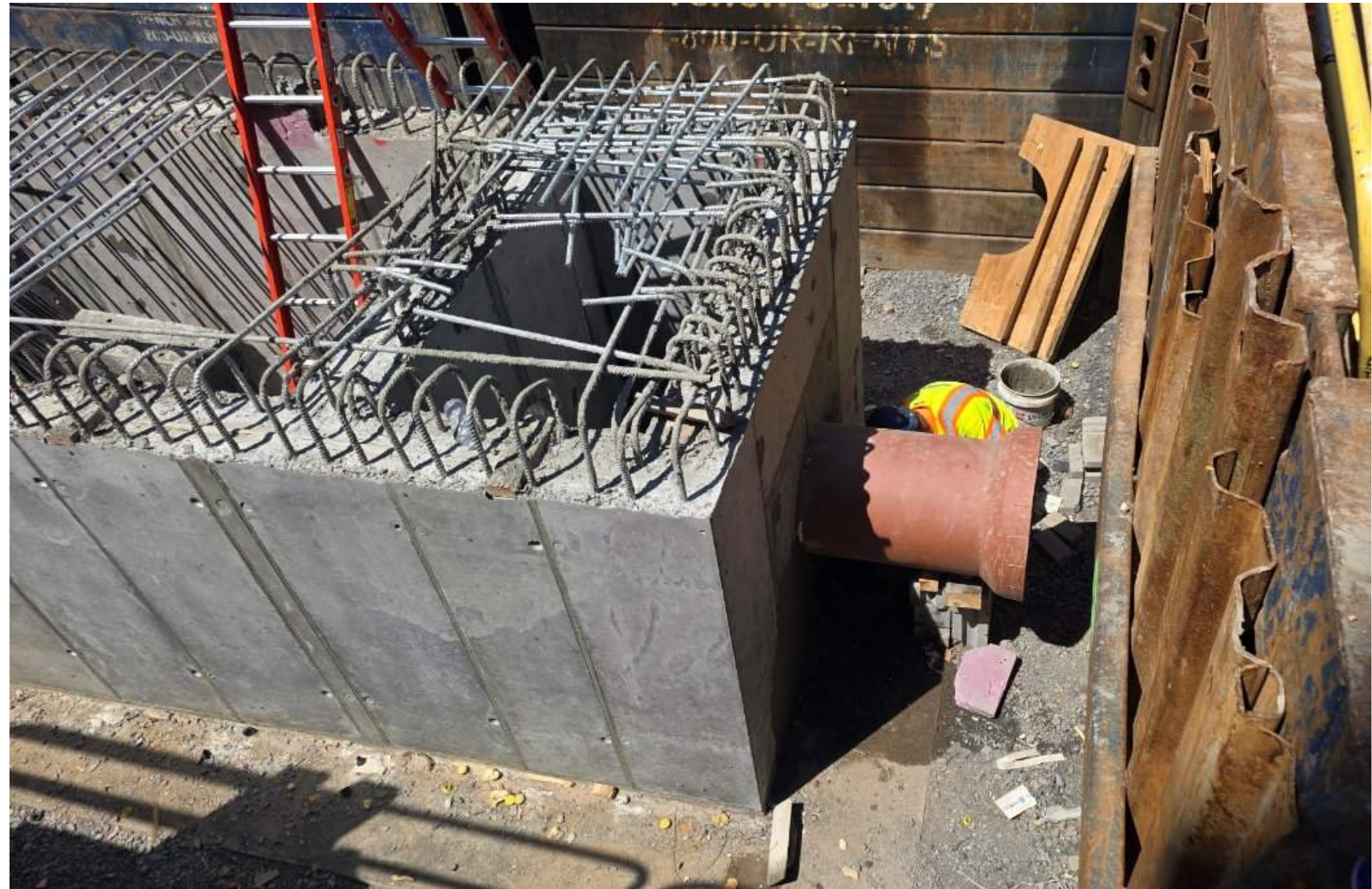
Concrete walls for tide gate chamber poured
