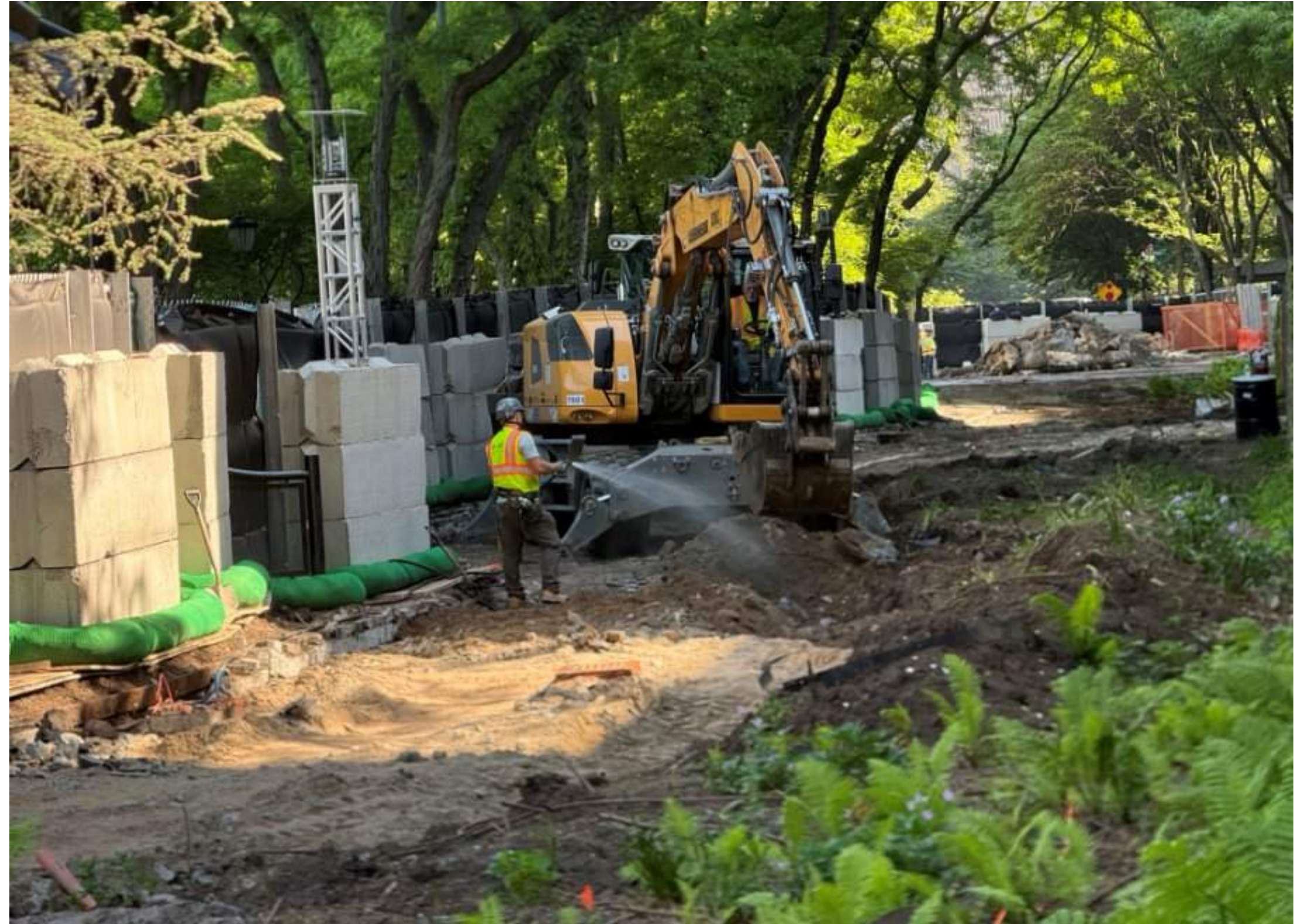
Surface Demolition at South Cove
