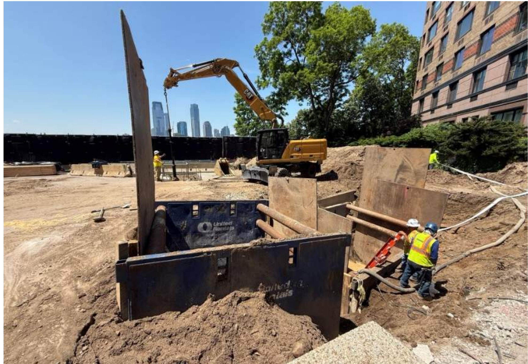
Test pit to identify subsurface utilities at proposed tide gate location
