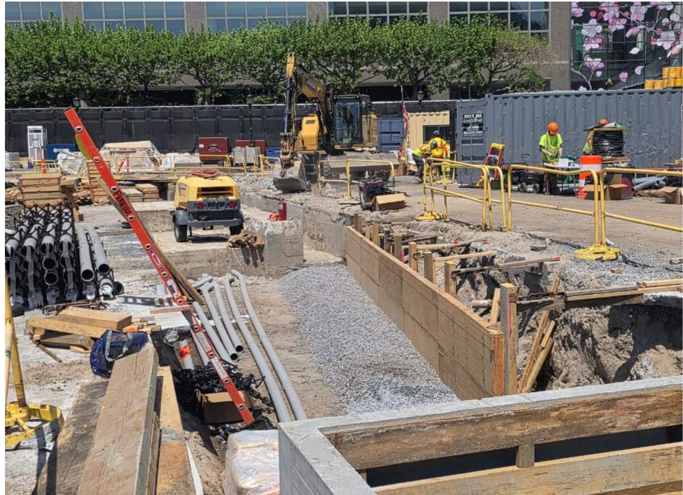
Trench for new ECS ductbank by Winter Garden
