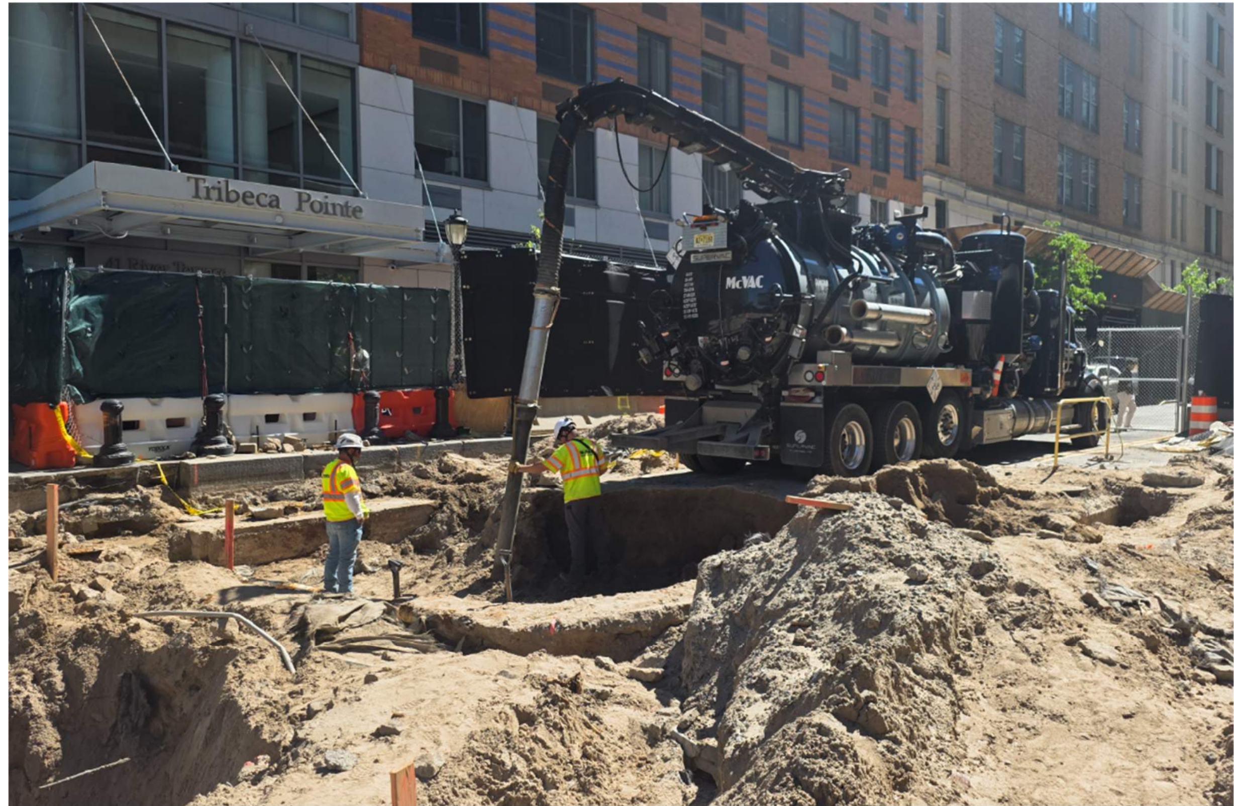
Excavating the electrical trench
