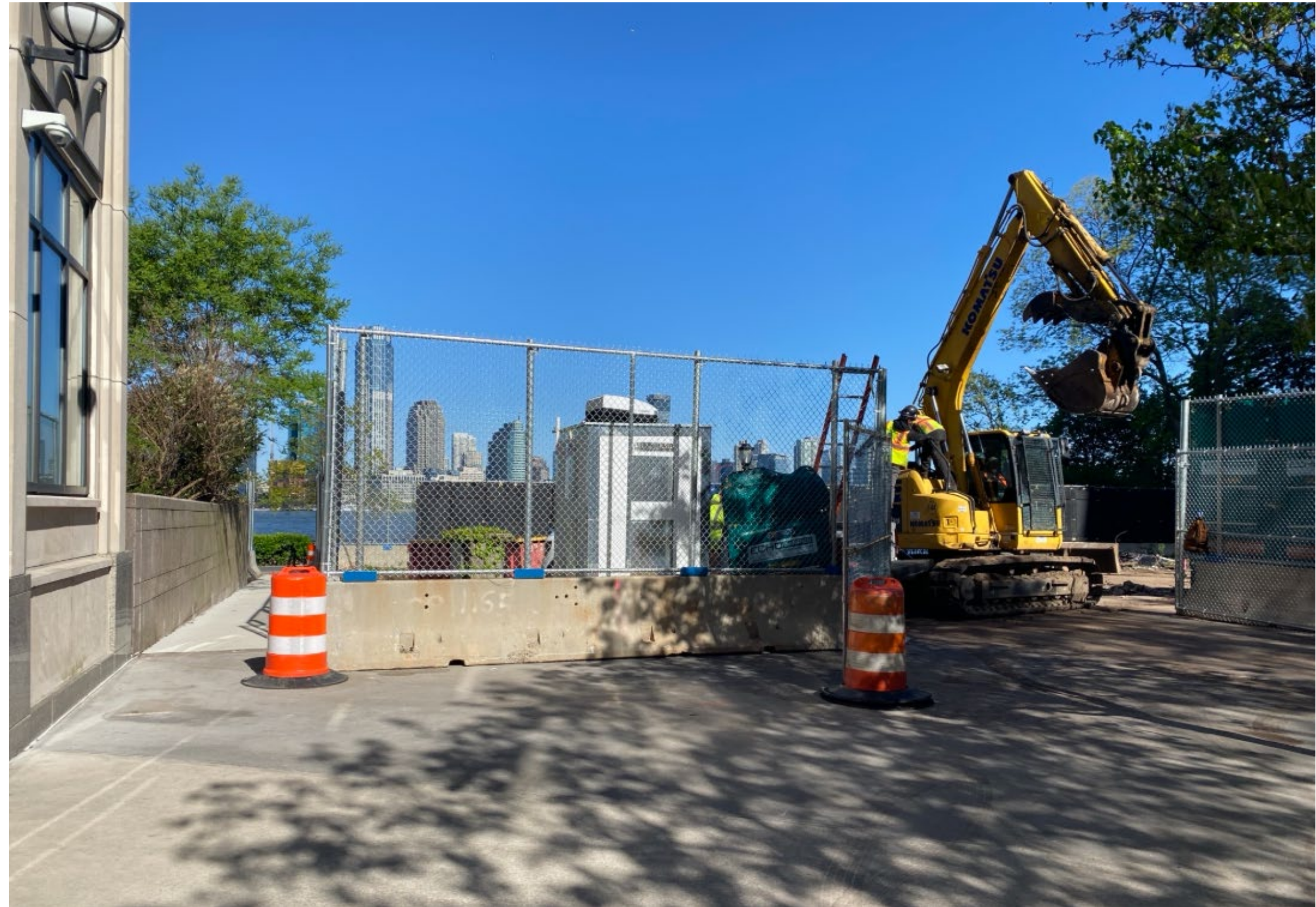
Surface demolition and pedestrian access
