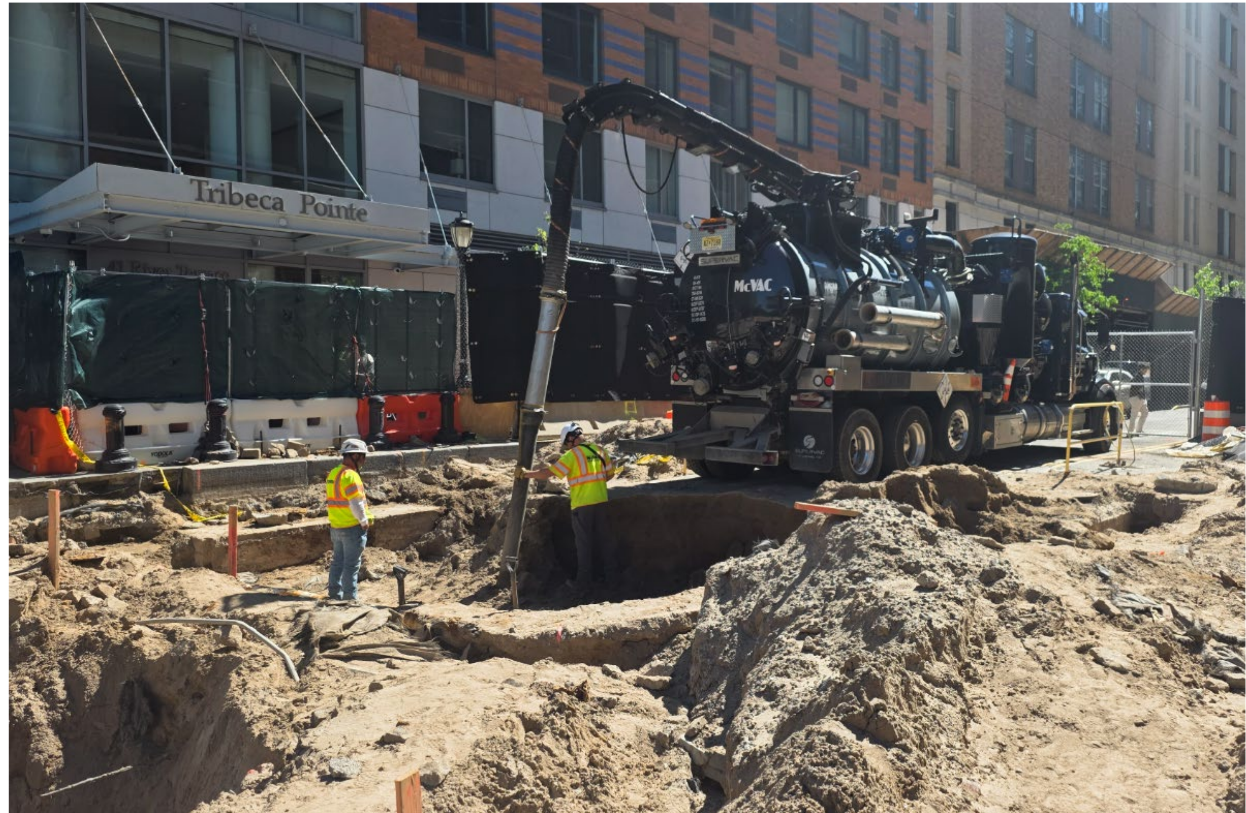
Excavating the electrical trench
