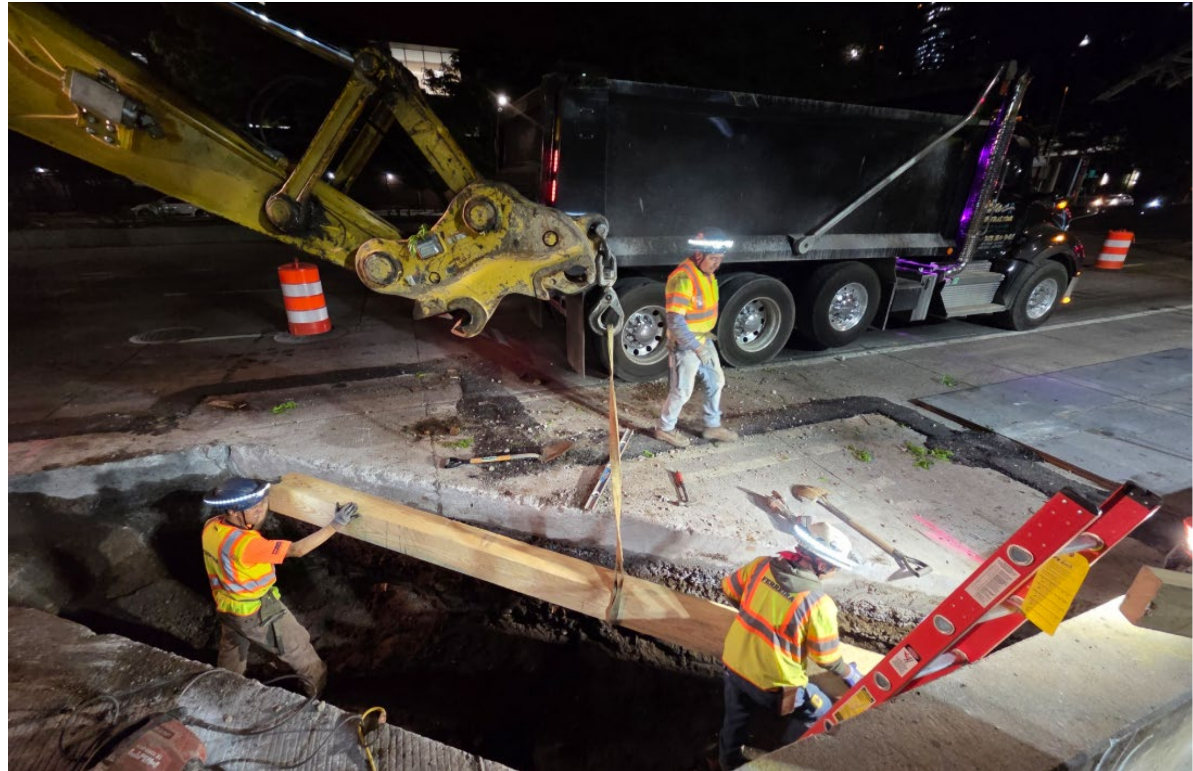
Nighttime work on West Street
