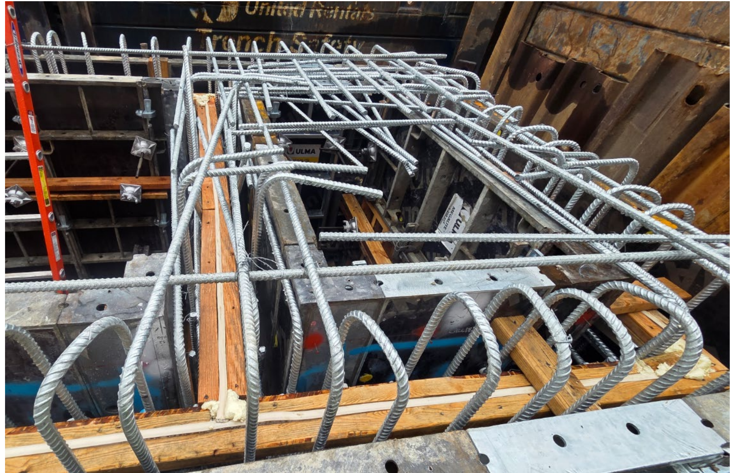
Installation of rebar for the walls and roof
