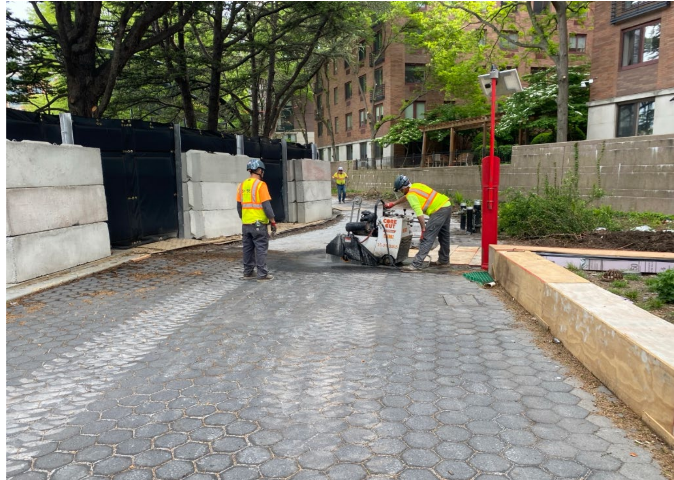
Surface Demolition at South Cove
