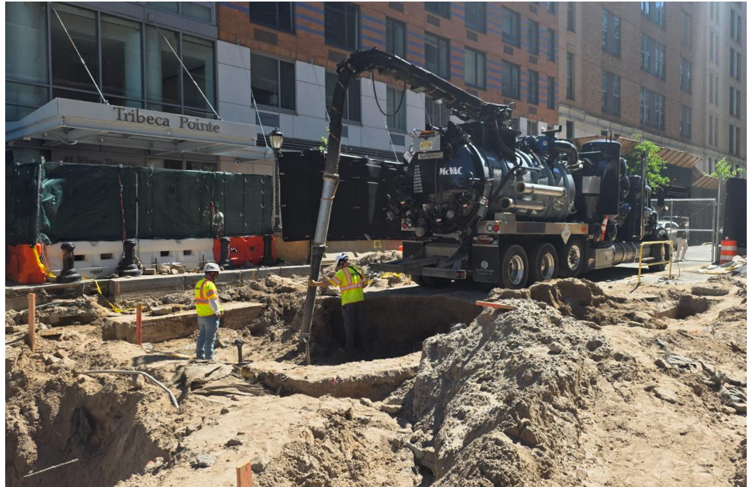
Excavating the electrical trench
