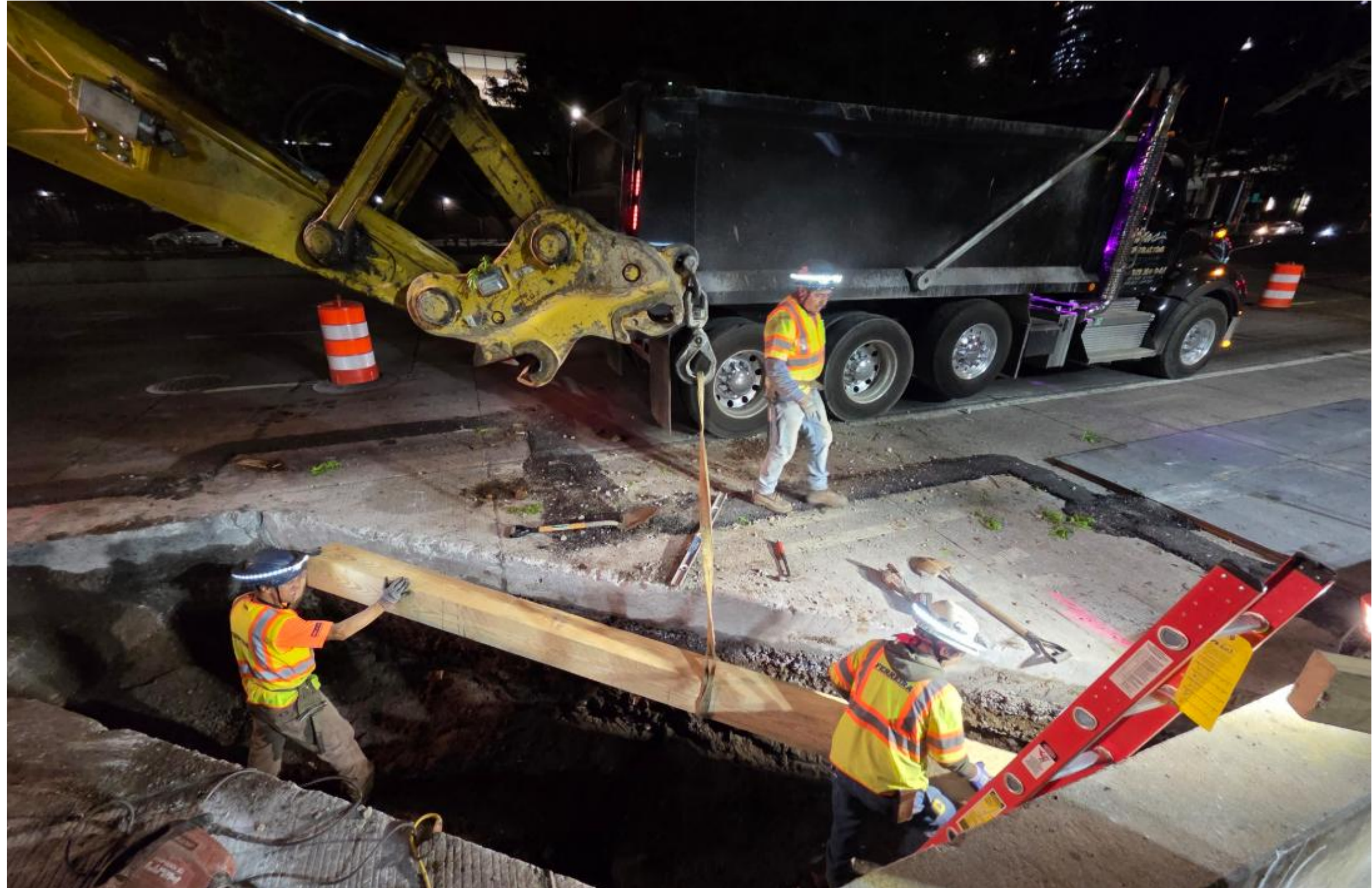
Nighttime work on West Street
