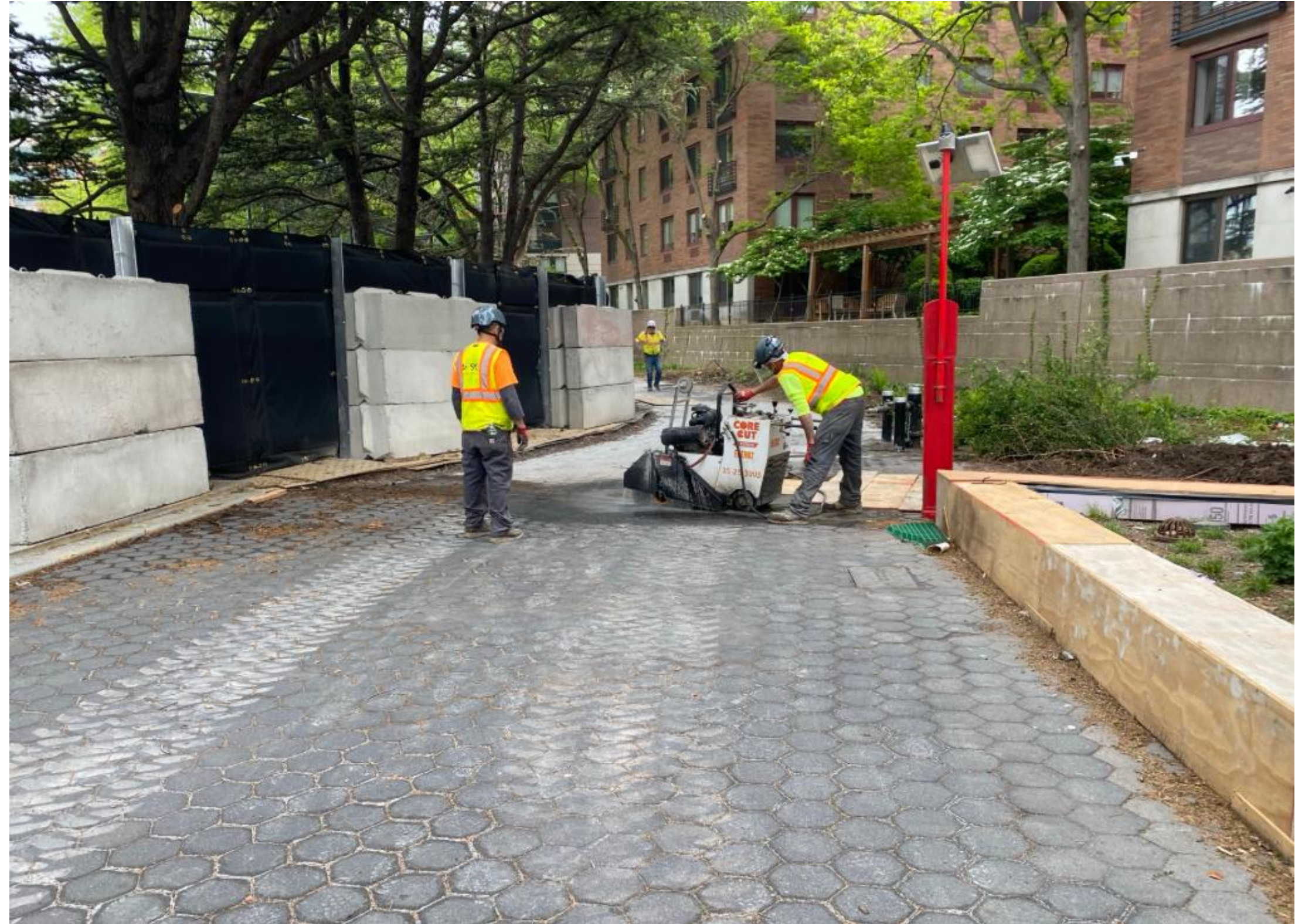
Surface Demolition at South Cove
