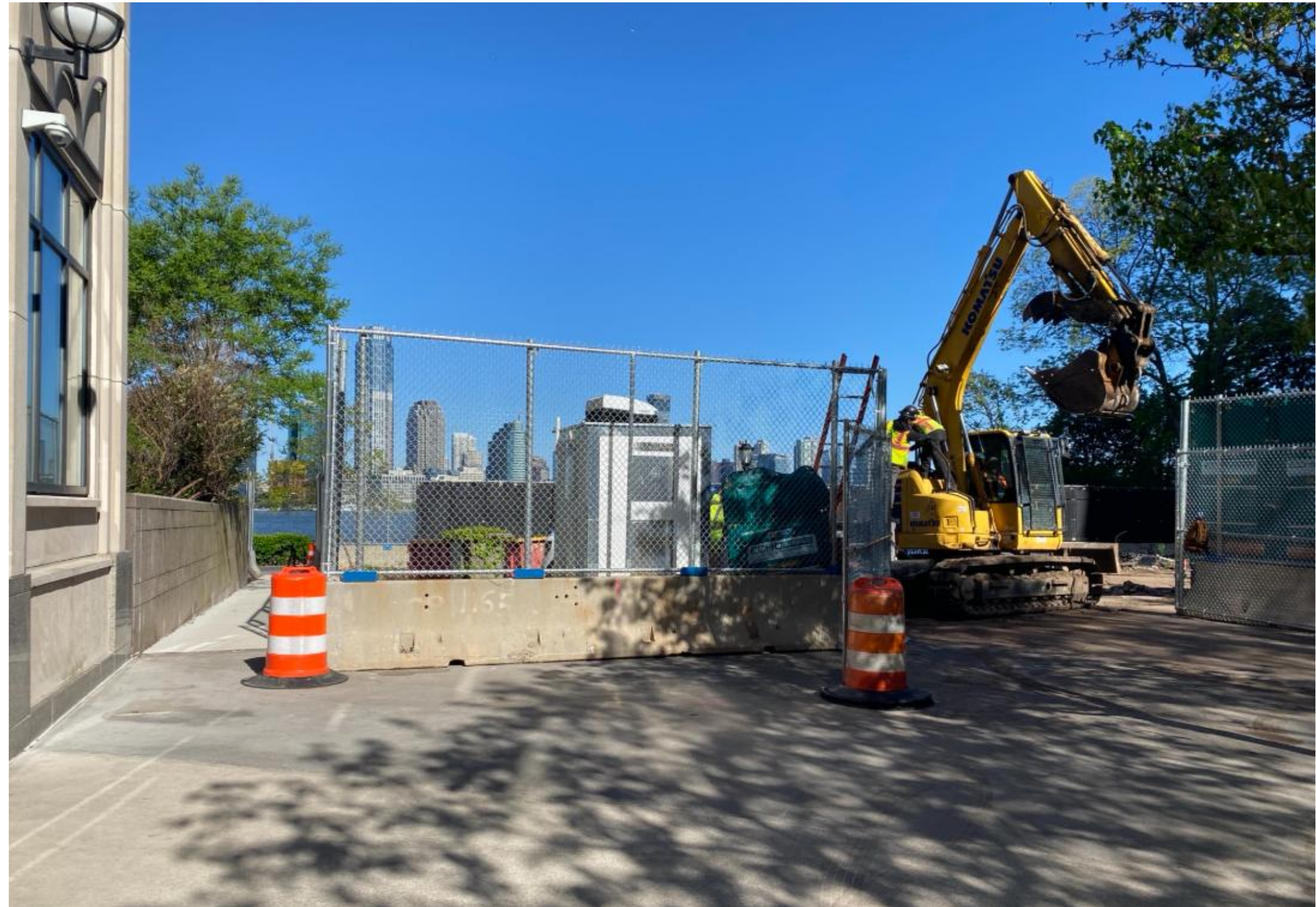
Surface demolition and pedestrian access
