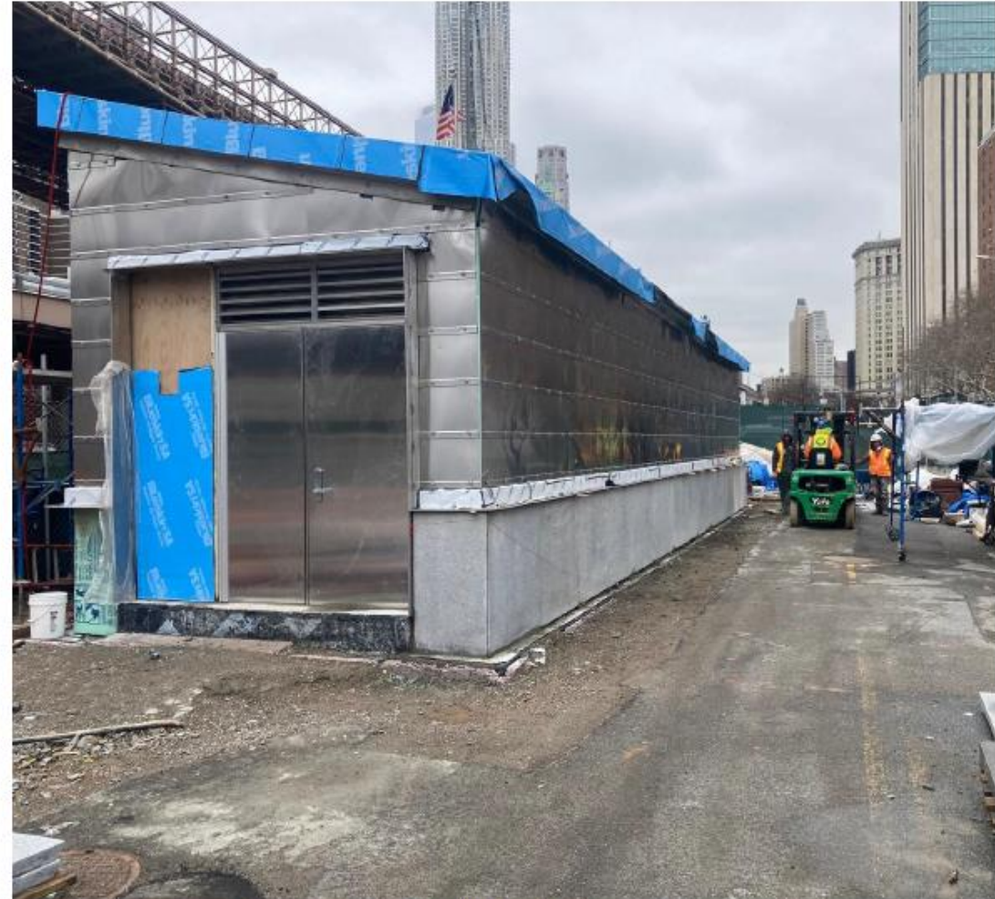
Construction of Interceptor Gate Building – March 2026
