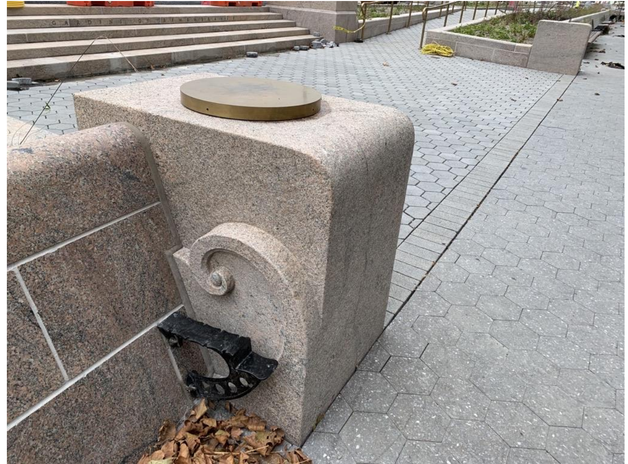
Newly furnished bronze cap installed on top of salvaged granite pier
