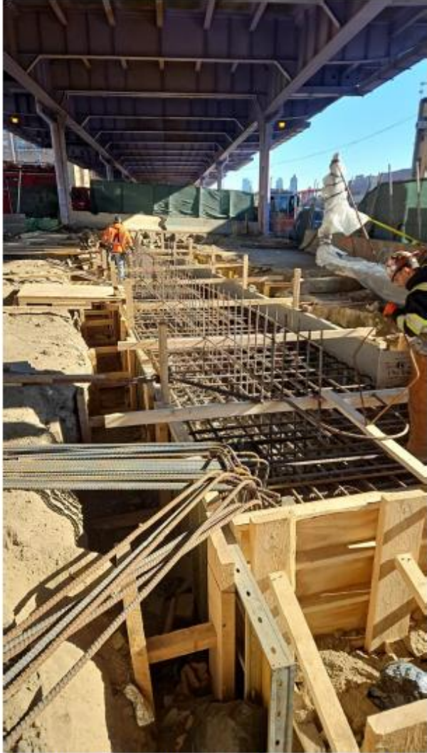
Formwork for floodwall footing under FDR Drive near Montgomery Street – January 2026
