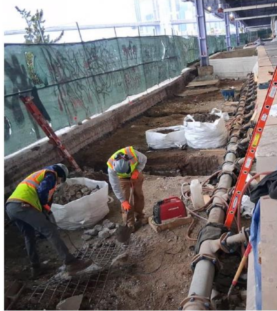
Utility work in coordination with Plus Pool – January 2026
