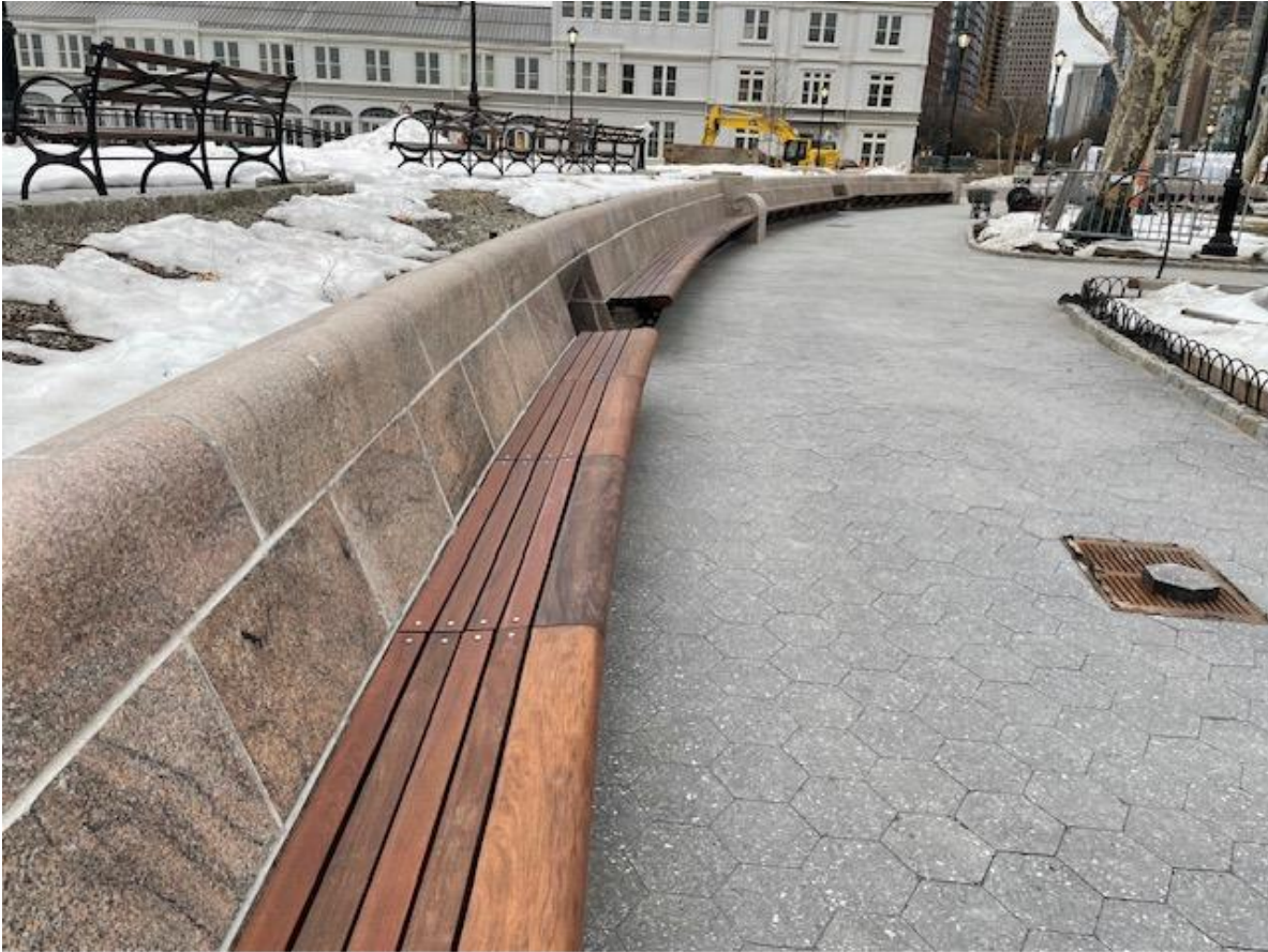
Refinished radial Granite-Backed Benches installed, awaiting new armrests
