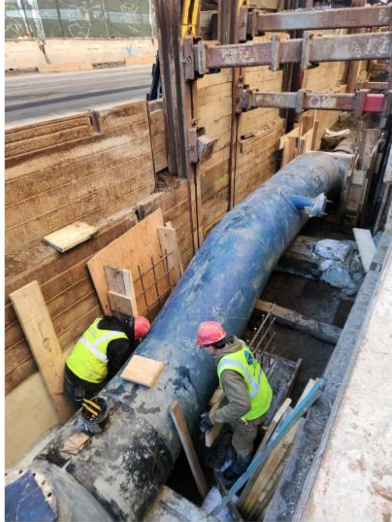
Trunk main installation in South Street – January 2026
