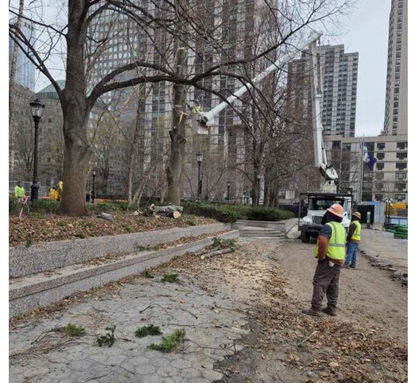
PUMPHOUSE PARK (Reach 5): Paver removal, trenching, tree protection and pruning, in preparation for utility relocation
