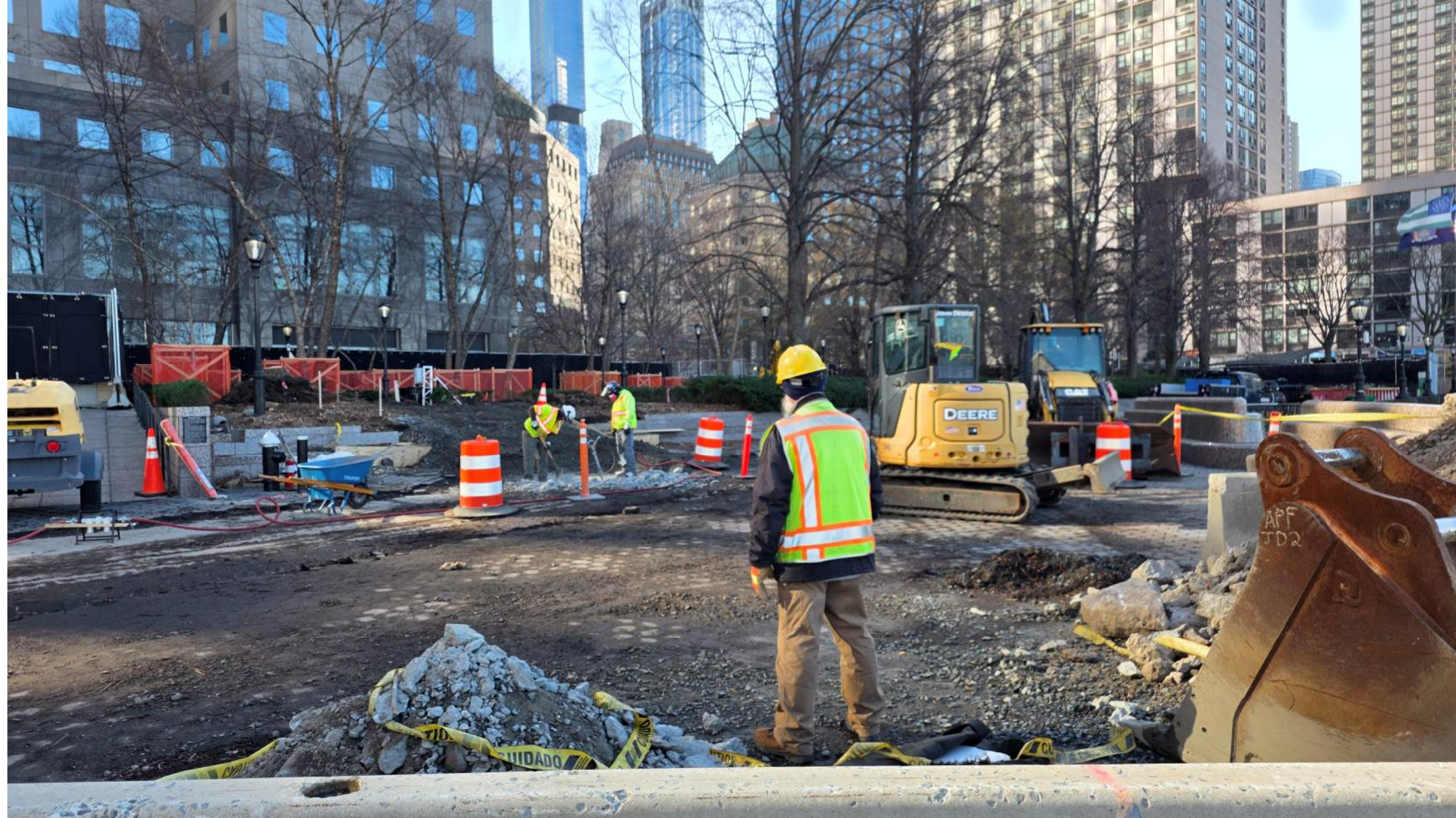
PUMPHOUSE PARK (Reach 5): Paver removal, trenching, tree protection and pruning, in preparation for utility relocation
