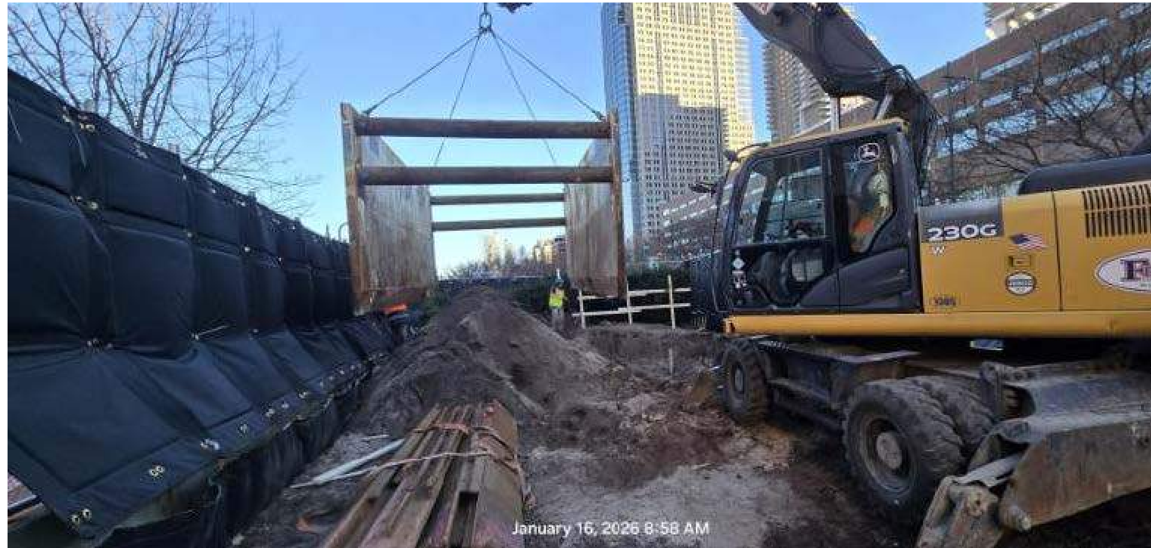
STUYVESANT PLAZA/HRPT (Reach 1): Capture work area, trench box installation, and demo
