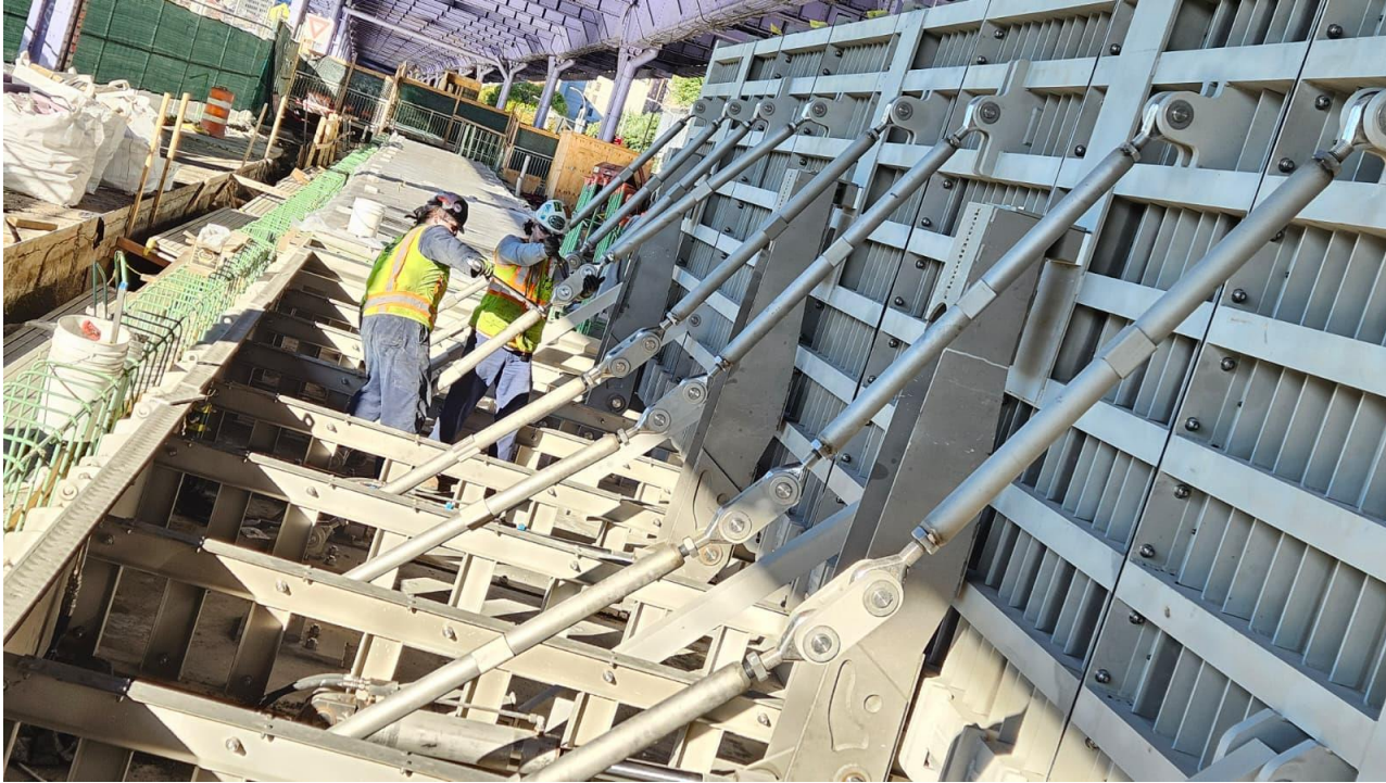
Flip up gate installation under FDR Drive – October 2025
