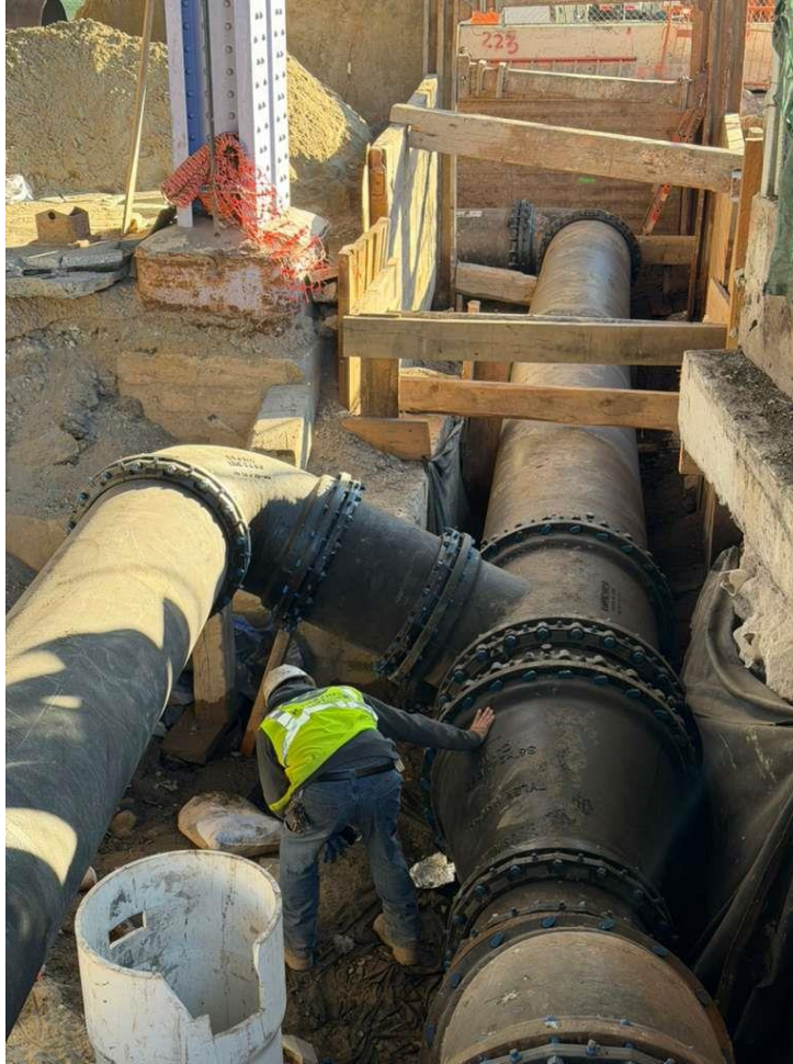
Trunk water main installation under FDR Drive – October 2025
