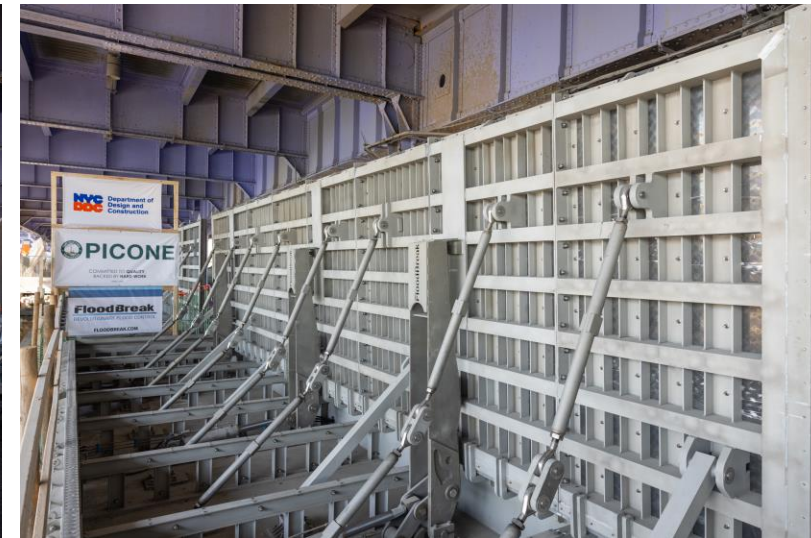
Flip up gate in open position – March 2025
