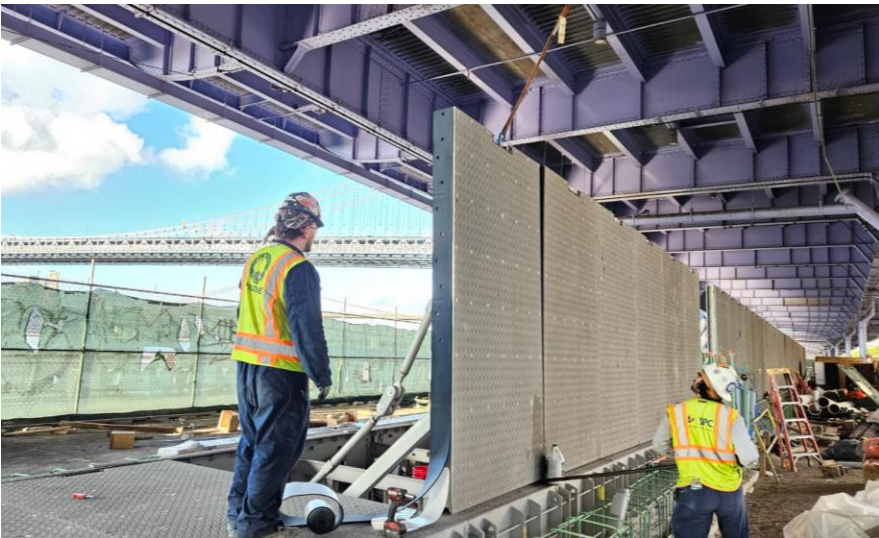
Flip up gate installation – September 2025
