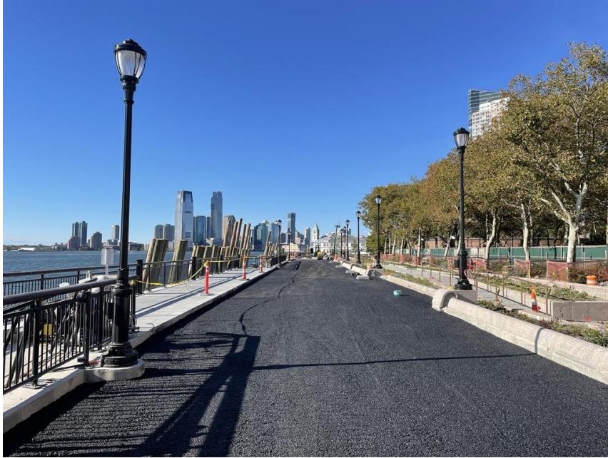
1. Asphalt Base Placed for Concrete Paver Field
