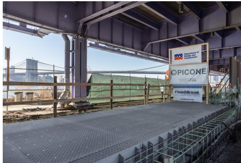
Flip up gate in closed position – March 2025
