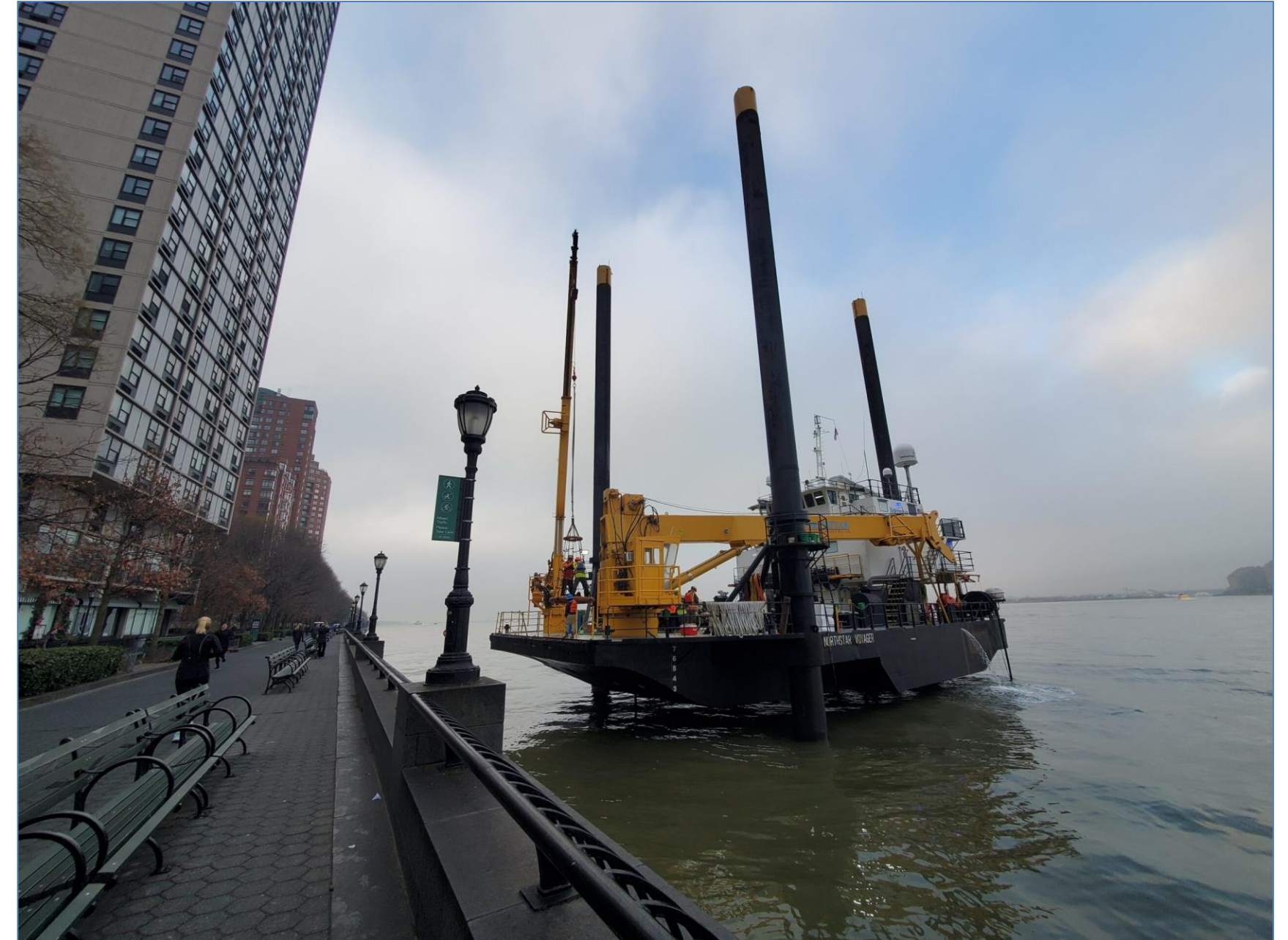
In-water geotechnical boring work taking place off Esplanade Plaza in February 2024.
