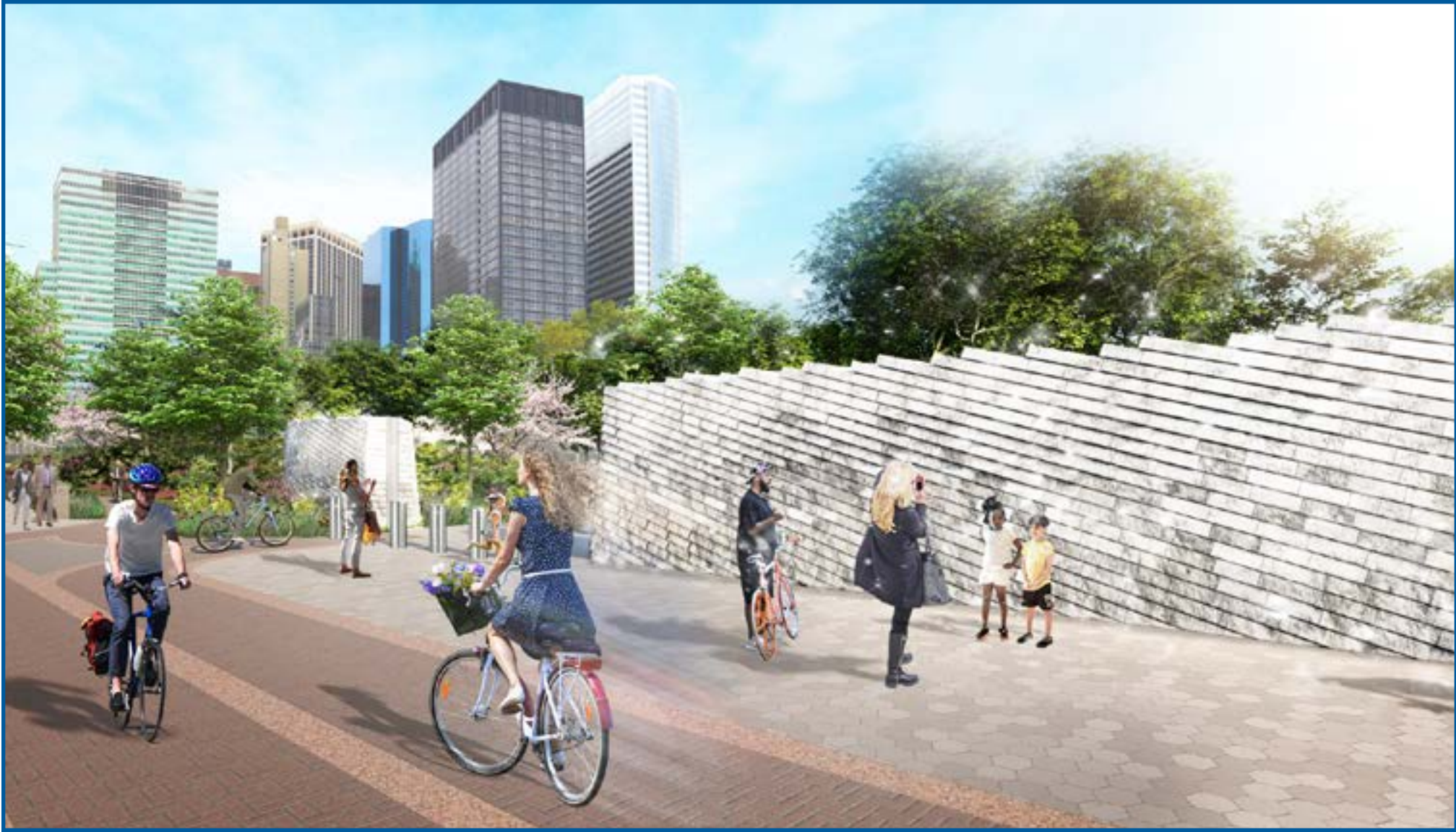
The exposed floodwall spanning the Battery Underpass is finished with an architectural stone veneer. New paving treatments improve pedestrian and bicycle circulation.
