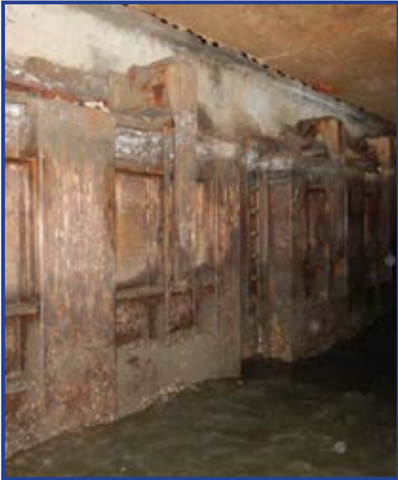
TIDE GATES Automatically close when the coastal surge is higher than the water level in the pipes
