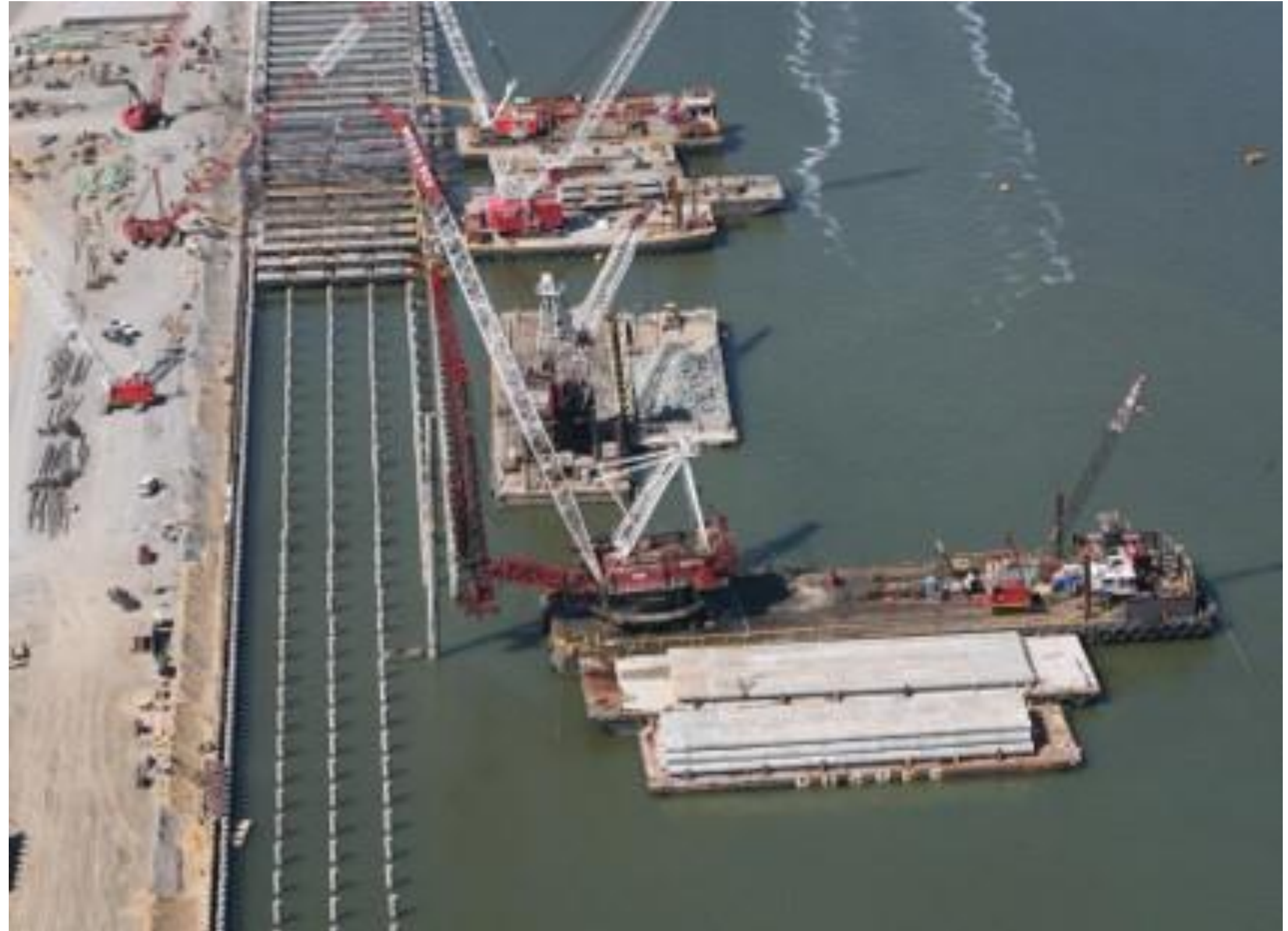
Platform Replacement along the North and South Esplanades will be assisted by equipment on barges
