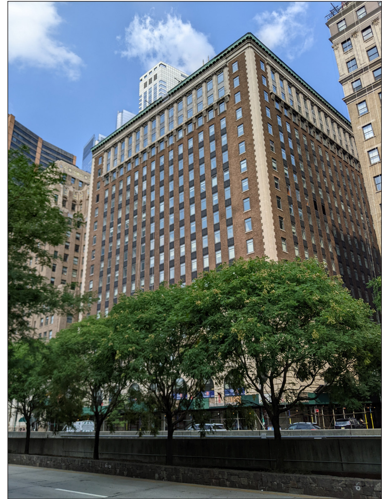
40 Rector Street, view northeast 22
