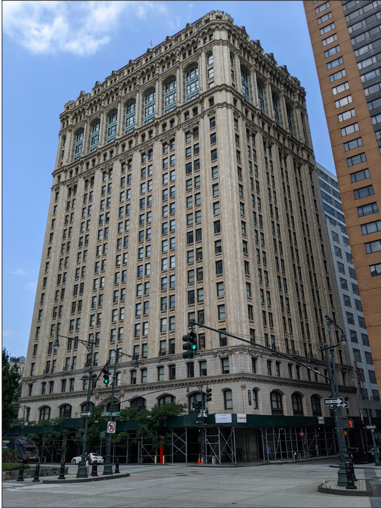
90 West Street, view northeast 19
