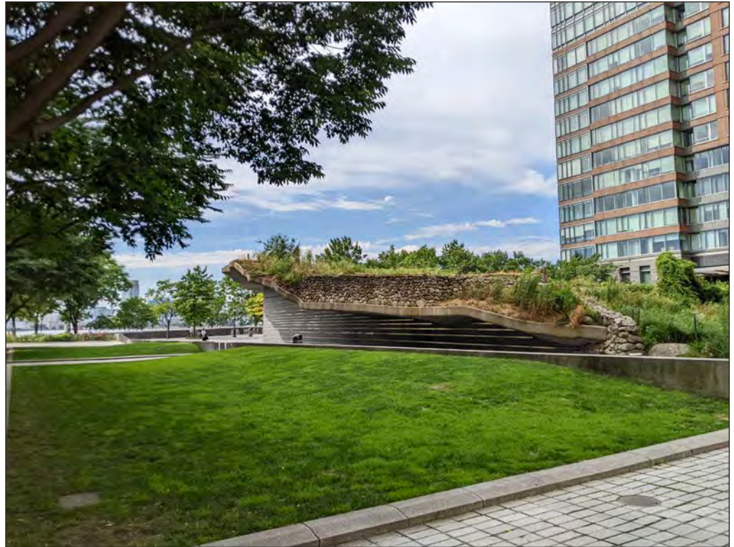
Irish Hunger Memorial, view northwest from North End Avenue 85
