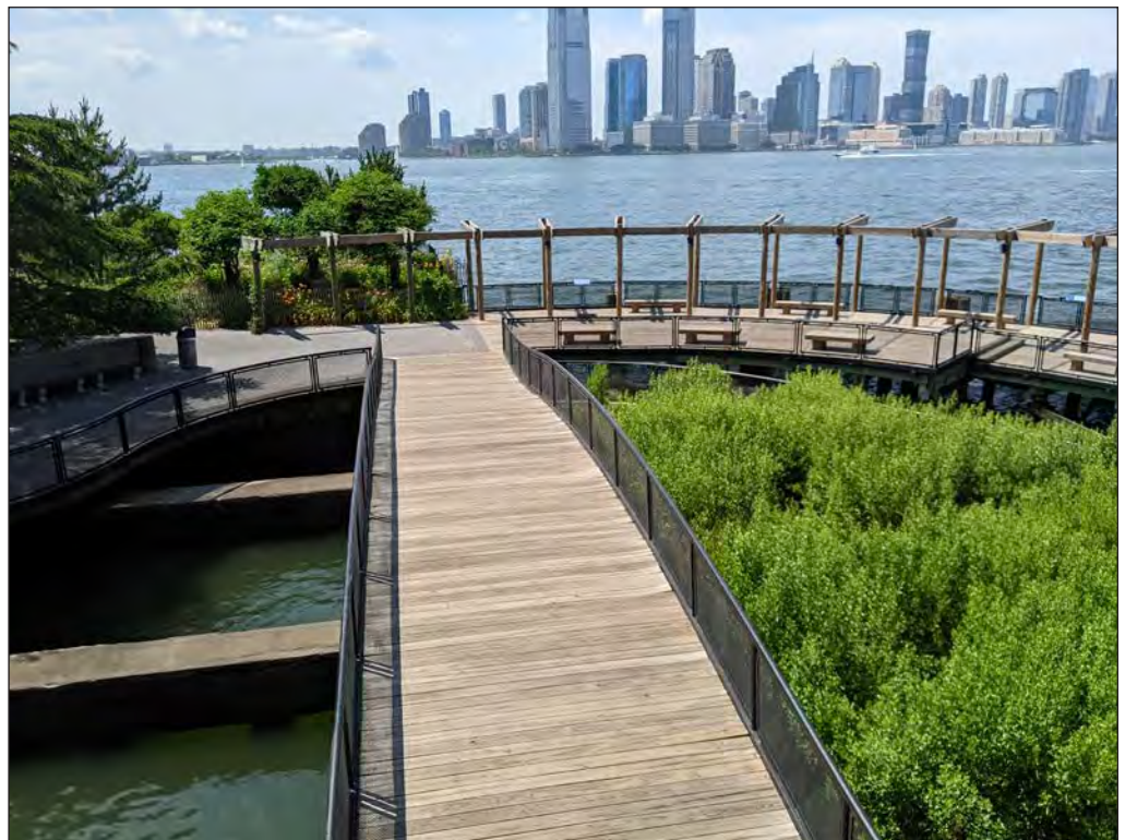
South Cove, view from lookout of island, bridge, and curved pier 46
