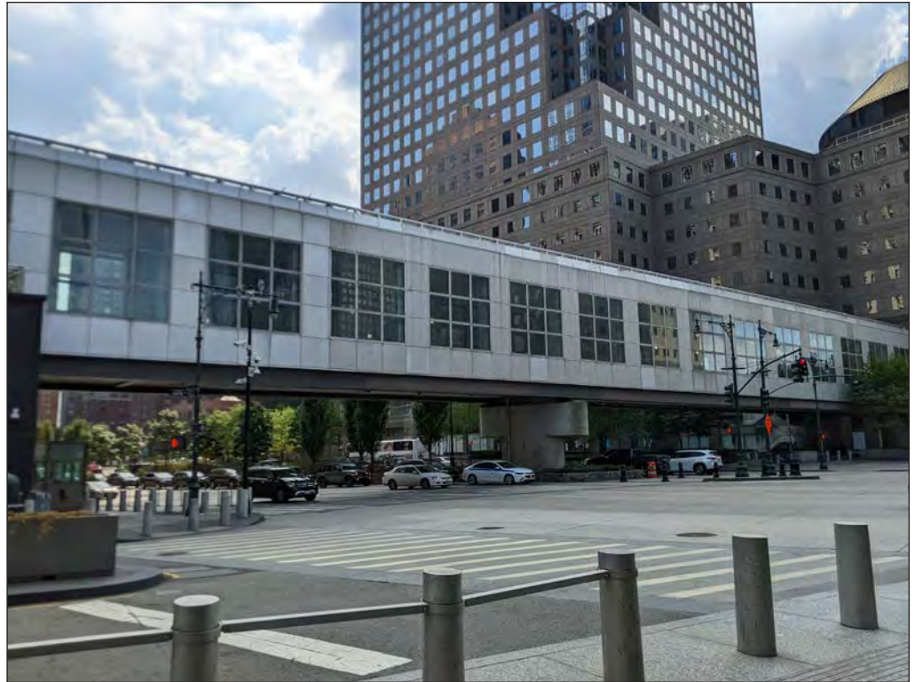
Liberty Street pedestrian bridge, view south on Route 9A (West Street) 3
