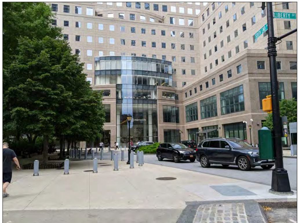
Brookfield Place entrance from South End Avenue, view north 74
