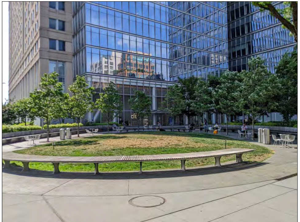
Citibank headquarters, view west of entrance plaza
