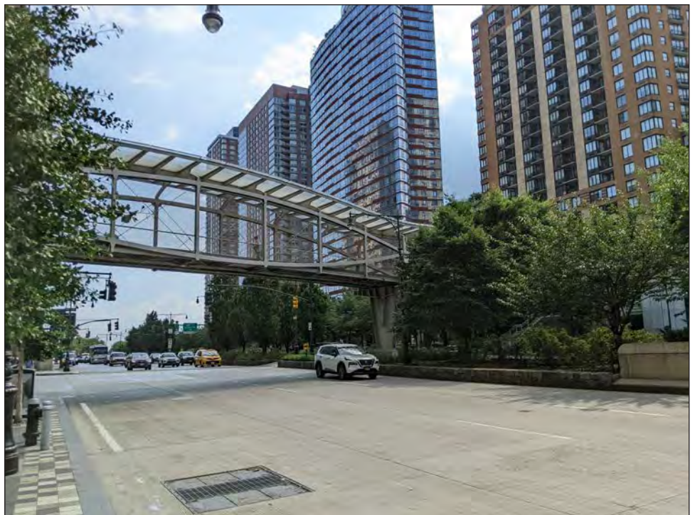
West Thames pedestrian bridge, view south on Route 9A (West Street)
