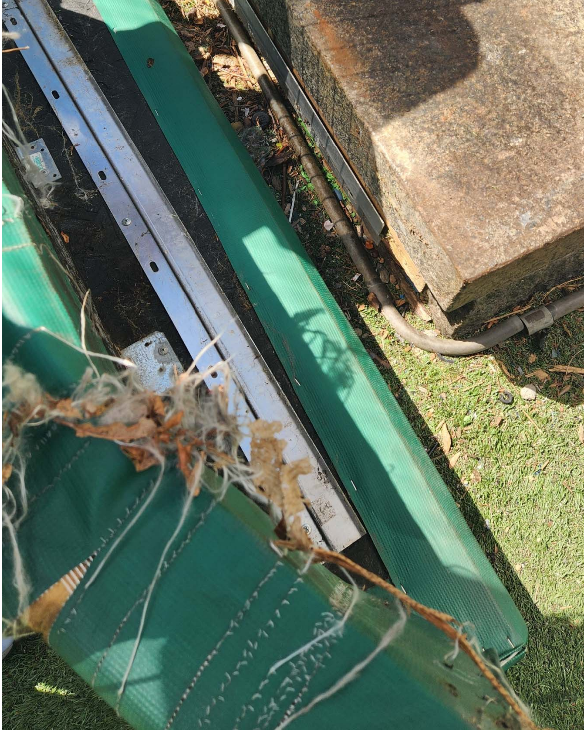
Horizontal pad with Z-bracket mounting hardware visible.
