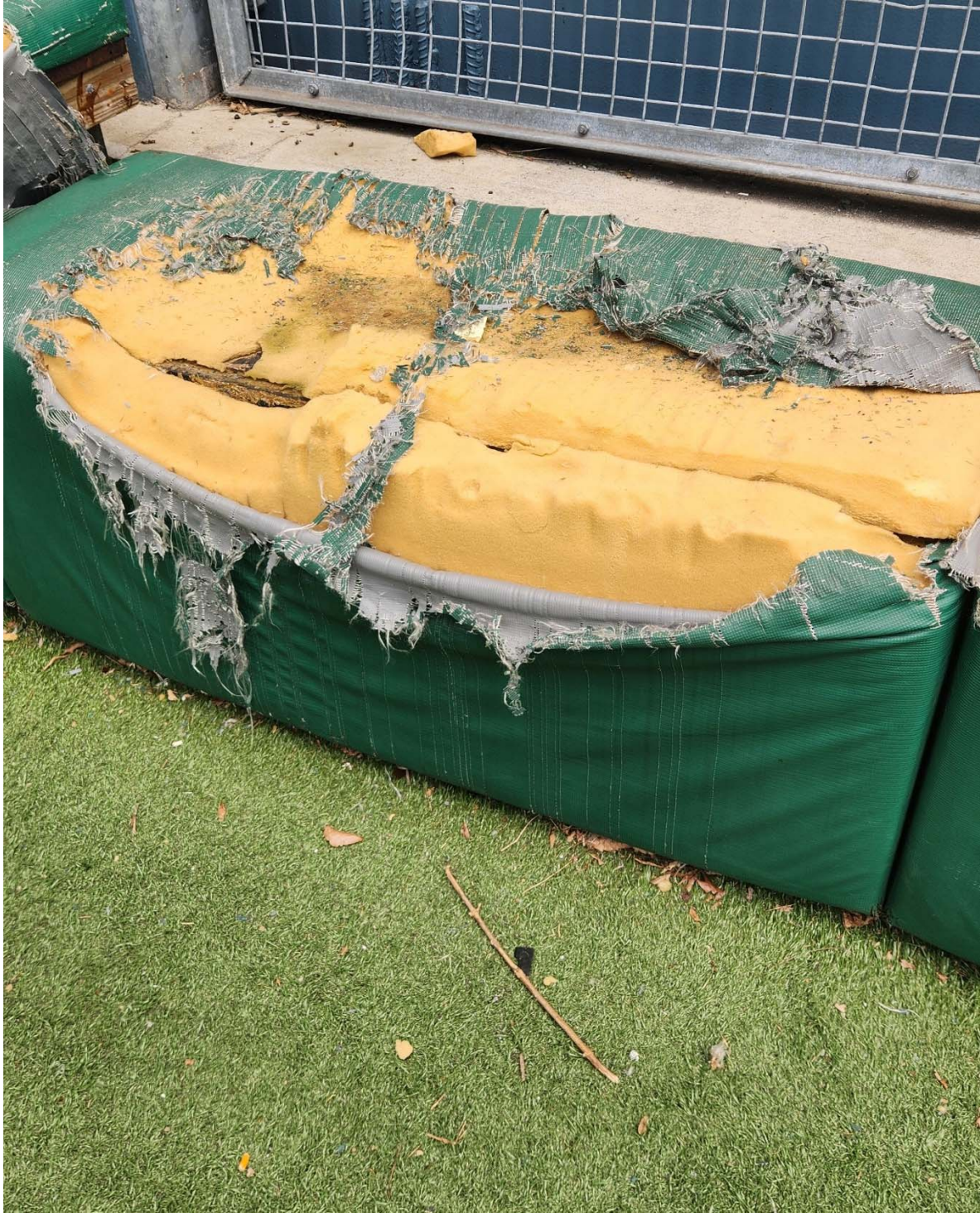
Wall barrier pad showing current level of wear.
