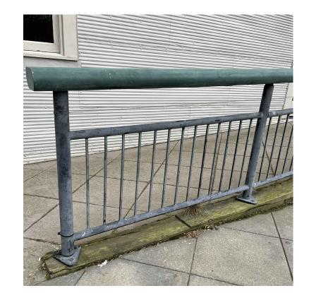
PHOTO NO.4 RAMP#1 HANDRAIL SUPPORT CRACKED
