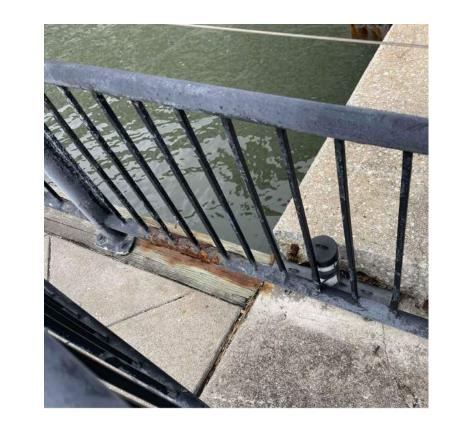
PHOTO NO.12 ENTRANCE RAMP NORTH CORRODED **HANDRAIL**
