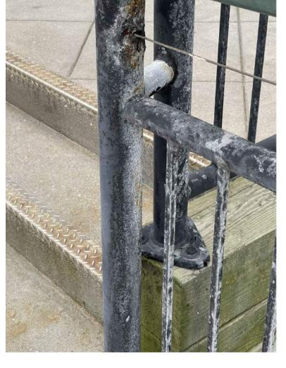
PHOTO NO.8 OPEN AREA #3 DETERIORATED HANDRAILS
