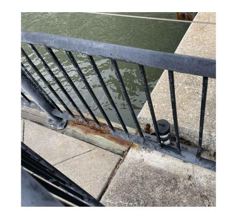
PHOTO NO.12 ENTRANCE RAMP NORTH CORRODED <u>HANDRAIL</u>
