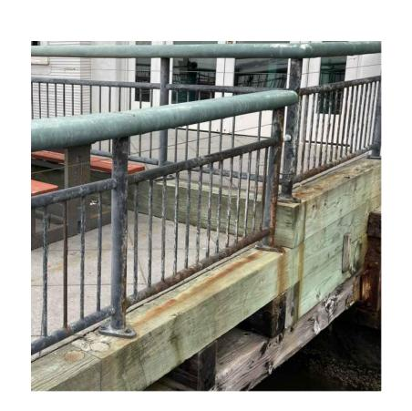
PHOTO NO.22 OPEN AREA #7 CORRODED HANDRAIL
