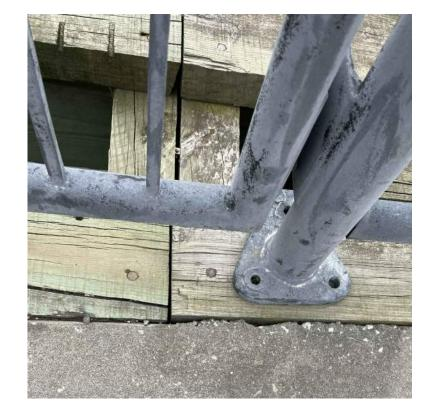
PHOTO NO.14 ENTRANCE TAMP SOUTH THREE BOLT MISSED IN TWO COLUMN BASE PLATES
