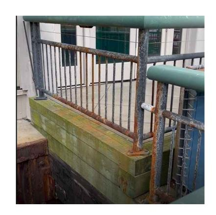
PHOTO NO.10 RAMP #2 CORRODED HANDRAILS
