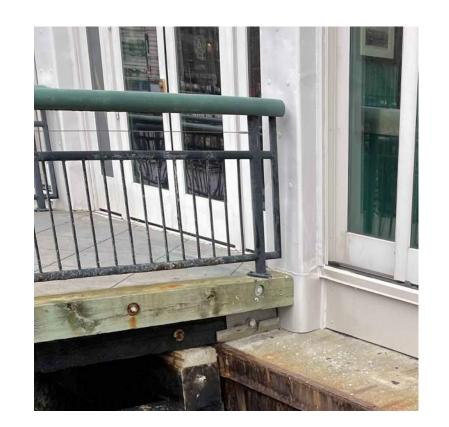
PHOTO NO.6 OPEN AREA #2 CORRODED HANDRAILS
