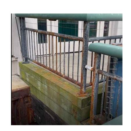
PHOTO NO.10 RAMP #2 CORRODED HANDRAILS
