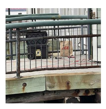
PHOTO NO.19 OPEN AREA #6 CORRODED HANDRAIL
