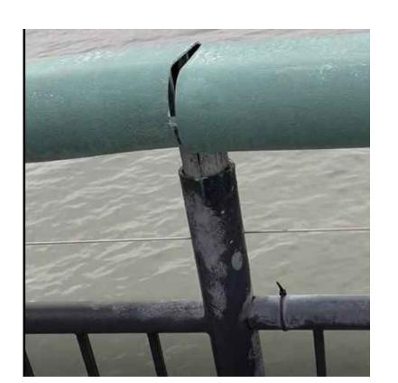
PHOTO NO.23 SOUTH PERIMETER HANDRAILS DEFORMED PIPE TOP RAIL
