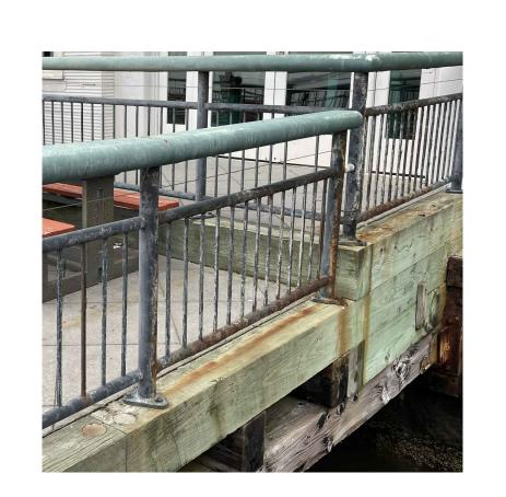
PHOTO NO.22 OPEN AREA #7 CORRODED HANDRAIL
