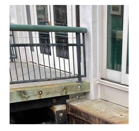
PHOTO NO.6 OPEN AREA #2 CORRODED HANDRAILS
