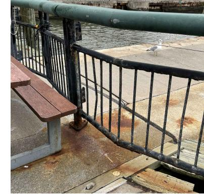
PHOTO NO.15 ENTRANCE RAMP SOUTH DAMAGED AND DETERIORATED HANDRAIL
