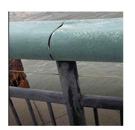
PHOTO NO.23 SOUTH PERIMETER HANDRAILS DEFORMED PIPE TOP RAIL NEAR FENDERS
