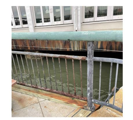
PHOTO NO.16 OPEN AREA #5 DETERIORATED HANDRAILS
