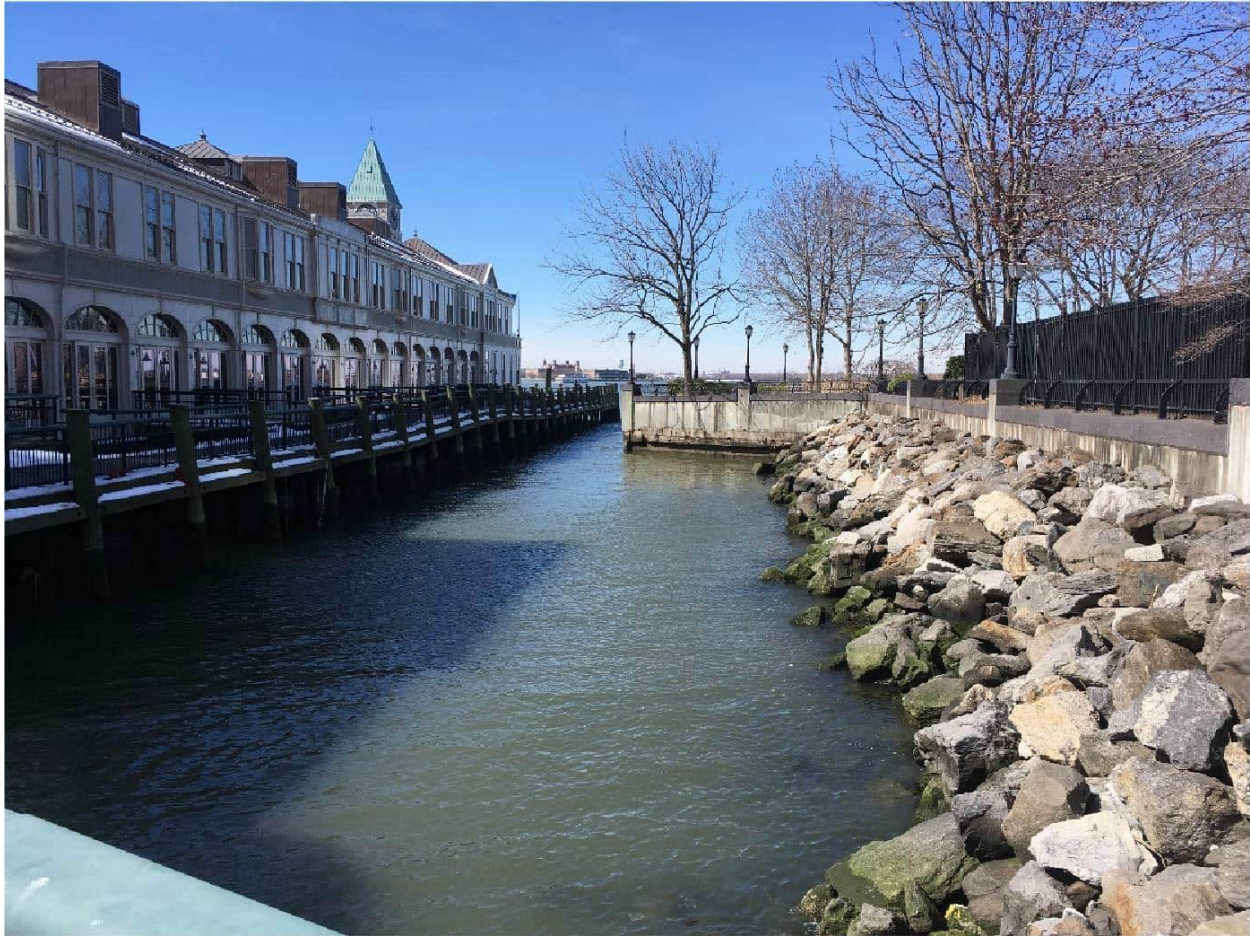
Figure 3.7-5: Photograph 1 – Looking west at the Pier A inlet. Note the unvegetated rip-rap shoreline of Wagner Park in the right side of the photograph
