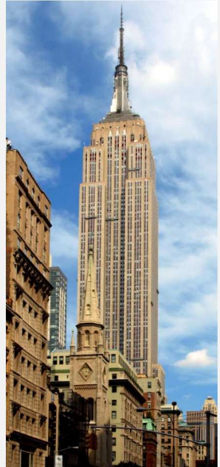
Figure 10: Empire State Building - New York, USA, 2015 88
