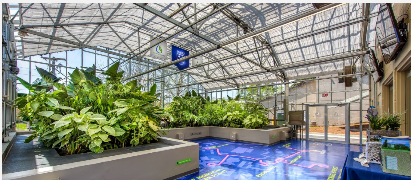
Figure 17: WaterHub at Emory University - Atlanta, USA 134
